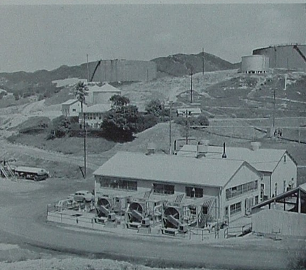
Above, the new equipment, using either gas or Diesel for fuel, requires giant fans to cool circulating water.
