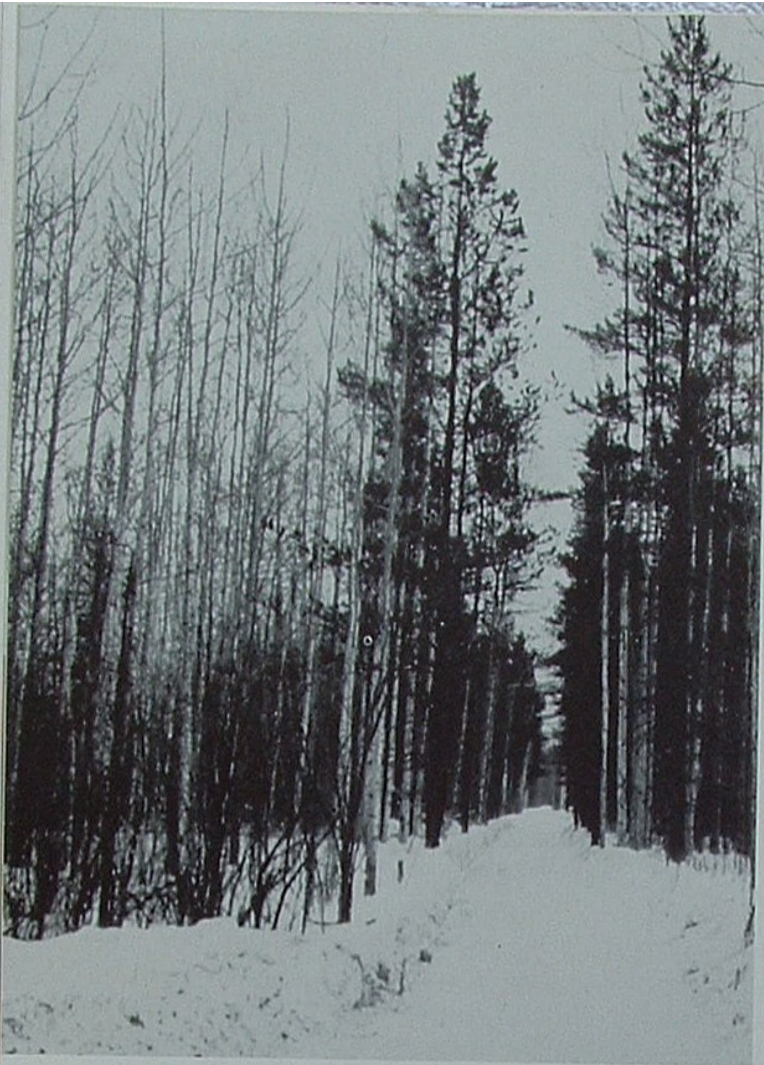
Winter roads are cut by bull-dozer through the tree-covered muskeg to admit trucks and exploration gear.
