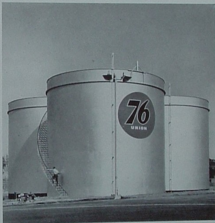
Four storage tanks, holding 10,000 barrels each, receive gasoline via 15 miles of pipe line from Los Angeles Refinery. Their floating roofs (below) rise and fall with stock levels, thus minimizing evaporation losses.
