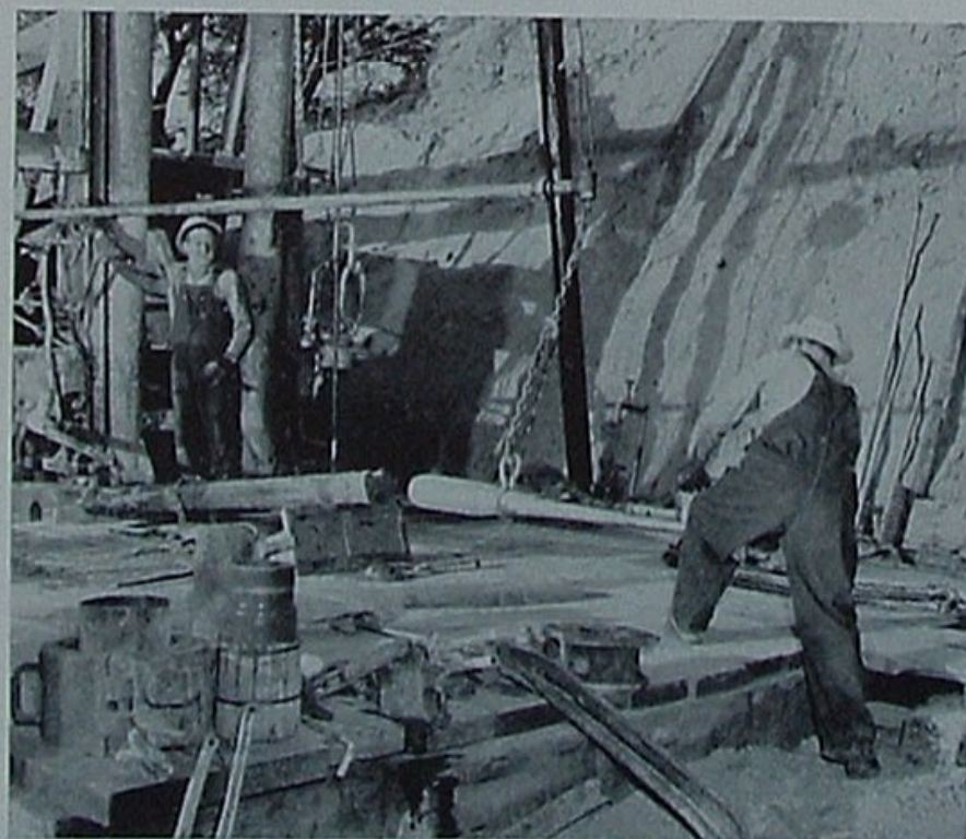
"Tool dressing" consists of flaring the white-hot end of a steel bit with the chain-supported ram (right).
