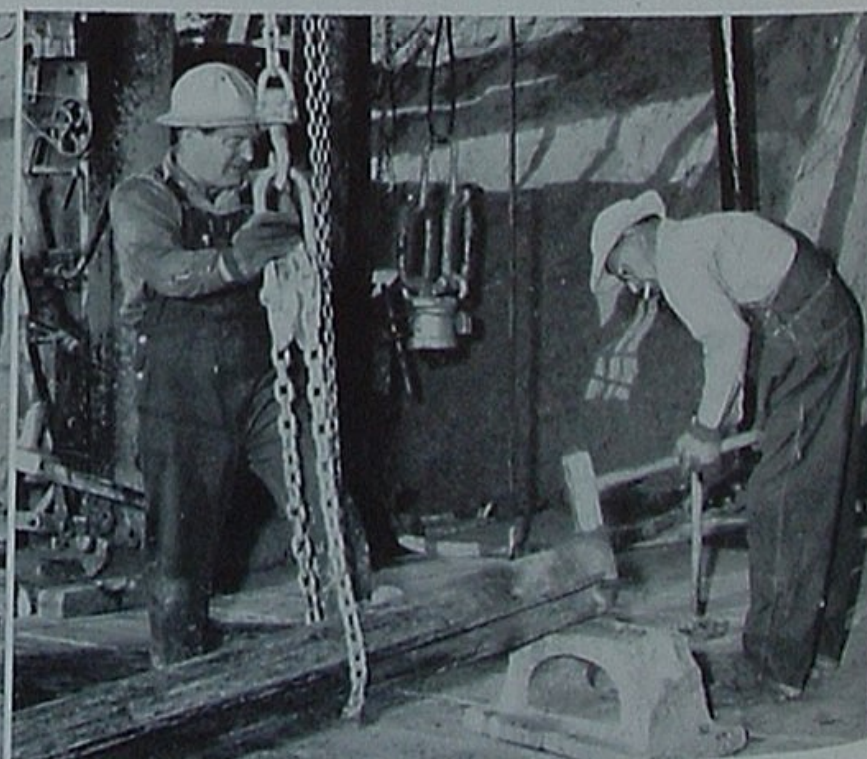
Cable toolmen W. R. Saunders (L) and I. E. Yarbo apply finishing touches to the bit with a deft sledge hammer.
