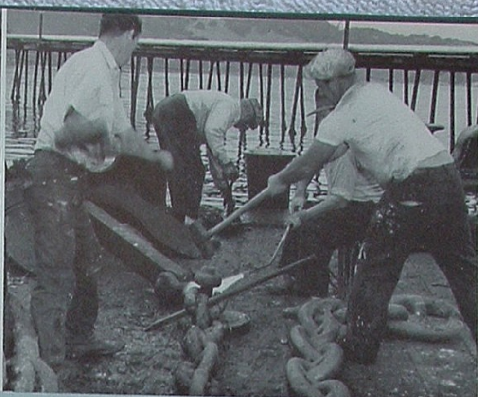
Above: On board a 100-ton servicing barge, workmen with sledge hammers and a torch reunite the locking anchor with its chain.
