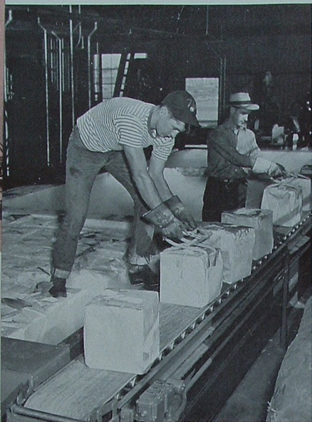
Plant storage for packaged ice is provided by three bins from which Jim Monk (left) and Dave Salmon are seen loading a conveyor. Workers avoid touching ice or inhaling its suffocating vapors.
