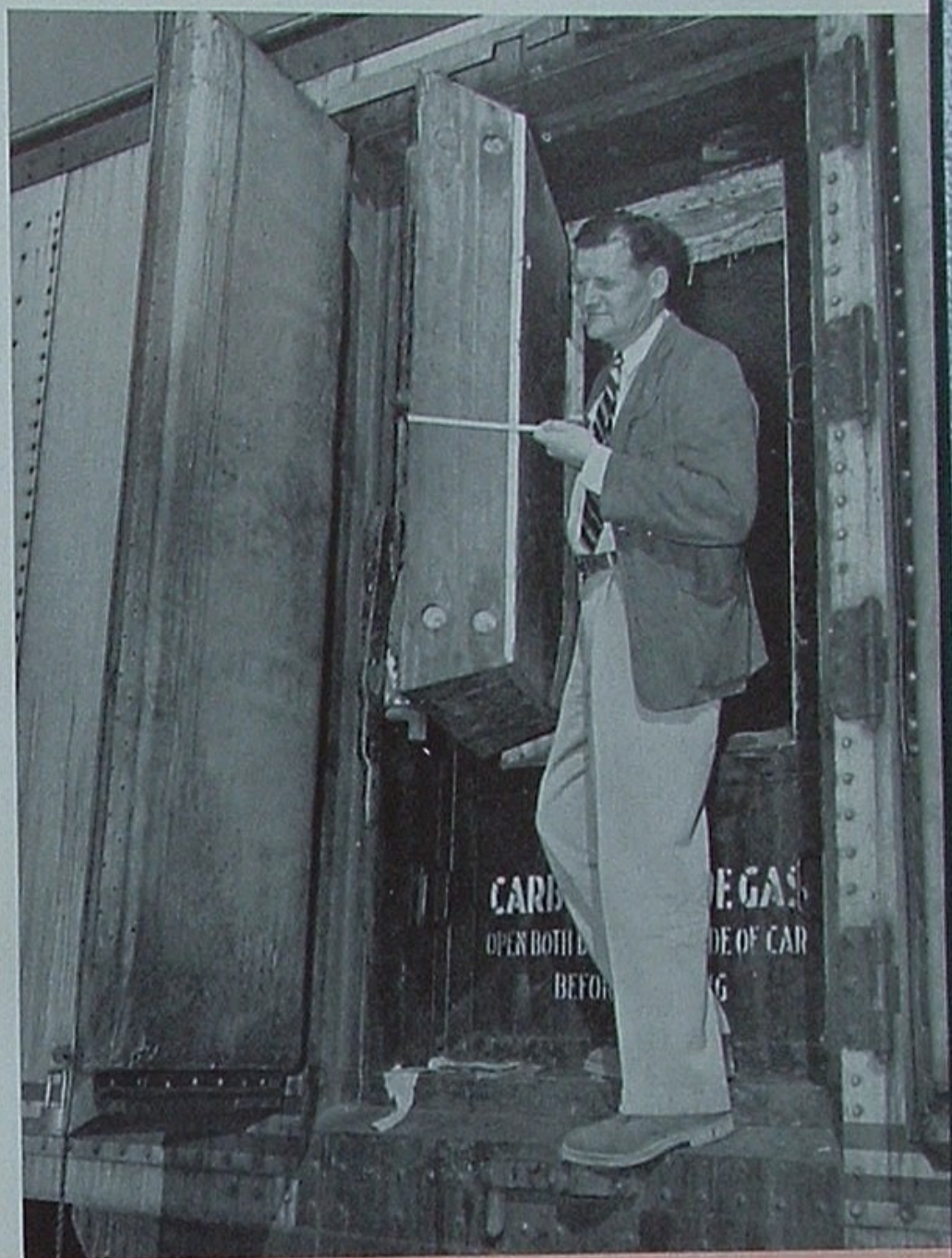
John Adams, field engineer, inspects double doors of special car used to transport dry ice throughout western states. Shipped in this manner, ice can be held to a daily shrinkage of one per cent.
