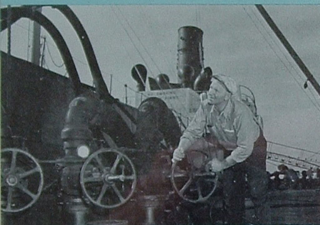
Above: Wharfinger Milton Selleck opens a 10-inch gate valve as the St. CLAIR begins pumping Poso crude to Oleum storage. Below: The ST. CLAIR is seen discharging the last of her crude cargo as a Liberty-type tanker loads refined products destined for Hawaiian Island delivery.
