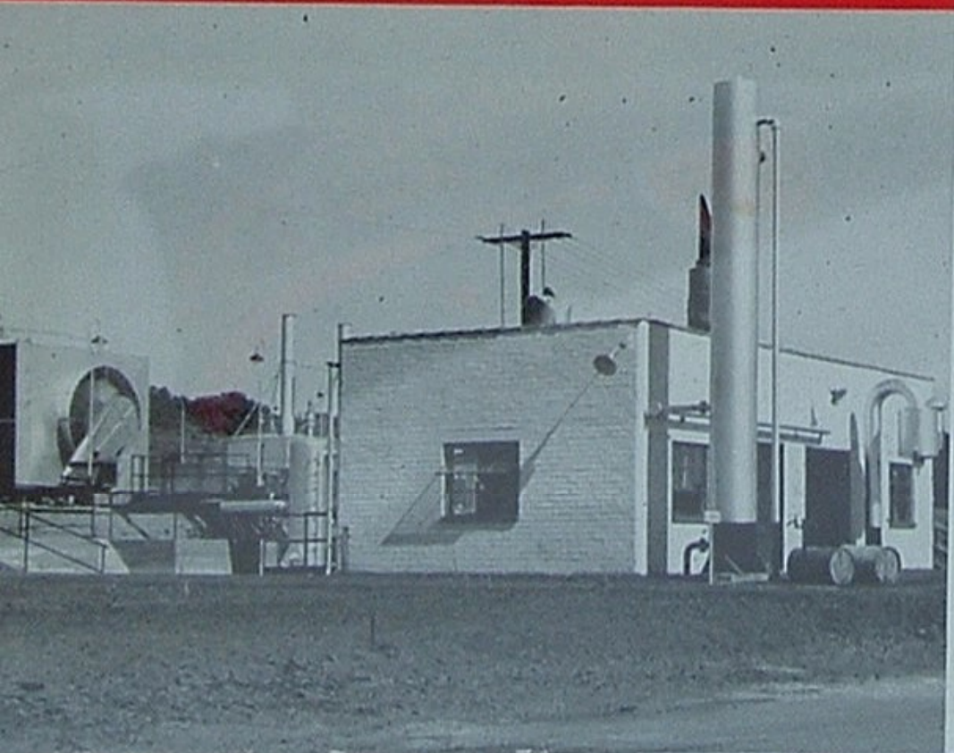
This unit in the Lompoc area pumps gas underground as a secondary-recovery method of holding back water and increasing the oil yield.
