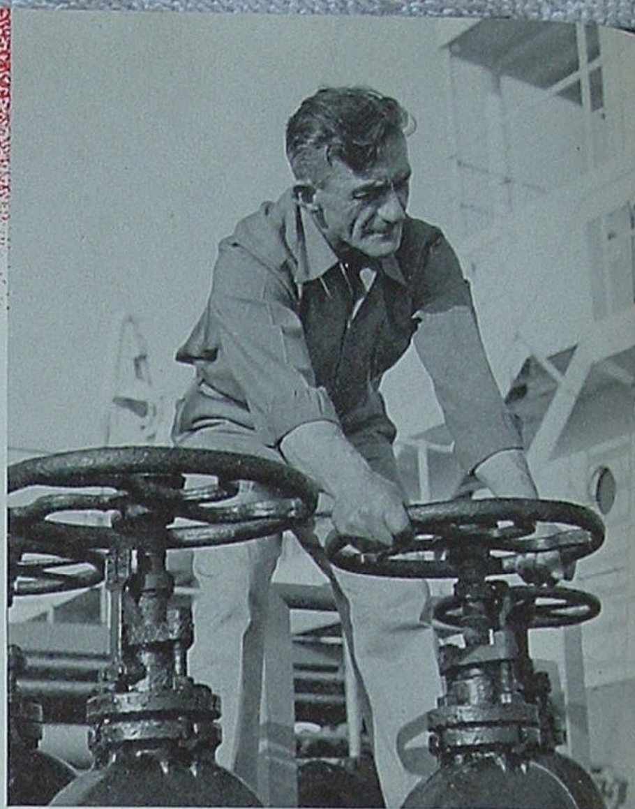
John Gordon opens the final valve preparatory to loading tanker oil compartments at pumping speeds up to 15,000 barrels an hour.
