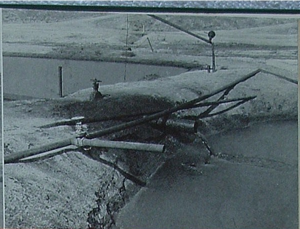
from the first sump, oil skimmings flow into a second sump for further settling and dehydration;
