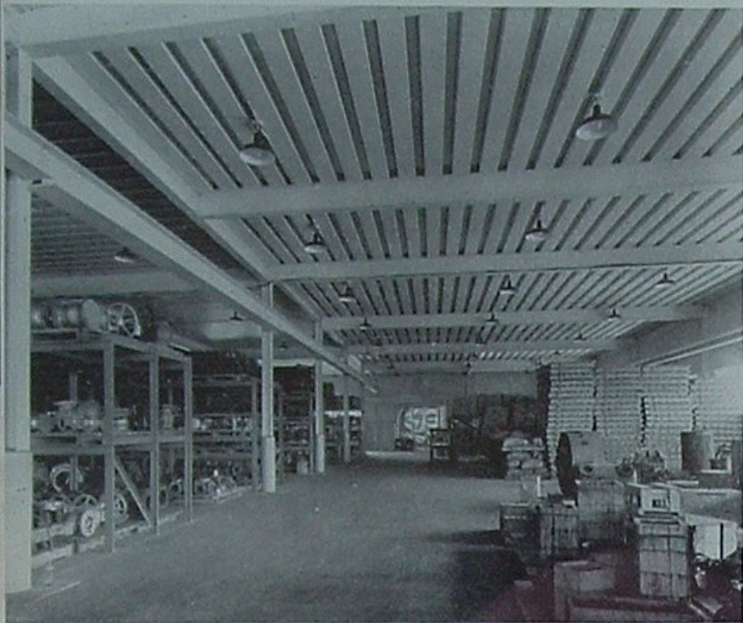
One of the new warehousing facilities recently completed as part of the extensive modernization program at Oleum Refinery.
