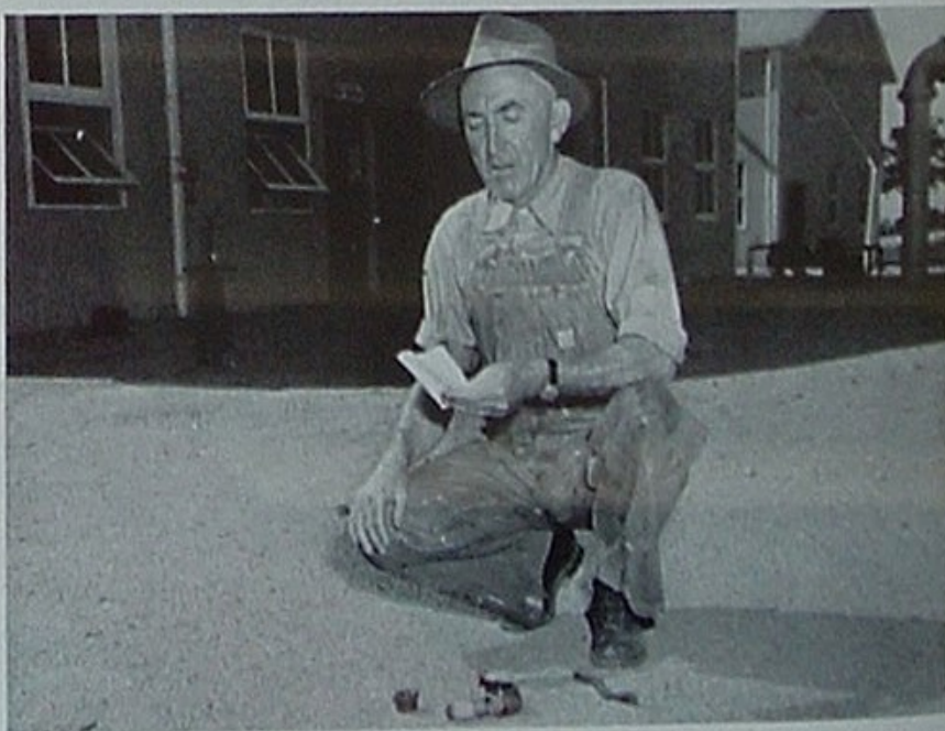
This particular leak report is picked up and read by Jack E. Harrington, senior engineer at Santa Margarita. He will immediately relay the report by telephone to a repair crew foreman.
