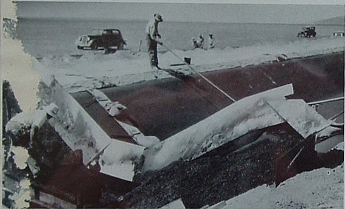
The asphaltic concrete used to line the canal contains Union Paving Asphalt of 60-70 penetration, is hot-mixed, hot-laid.
