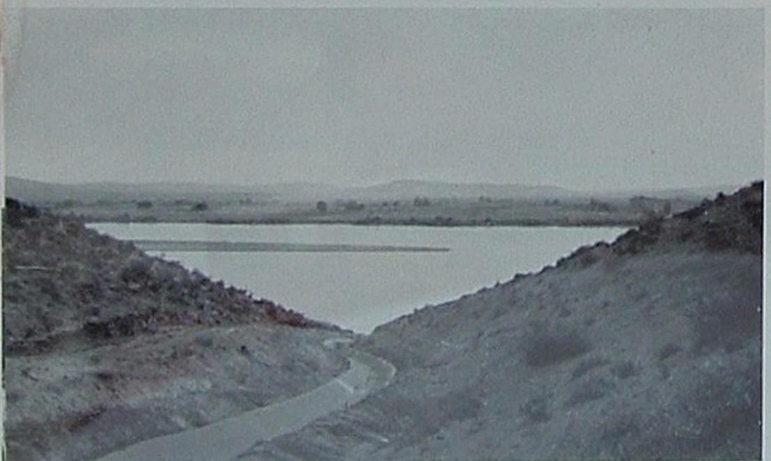
The completely-lined canal loses practically no irrigation water through seepage, discharges any surplus into the Columbia.
