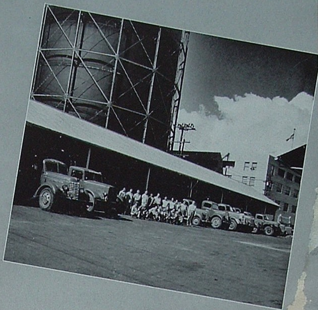
Drivers and Plant Employees, above, remember Pearl Harbor. During raid, they worked night and day delivering gasoline to the Army and Navy, despite bombs, shell bursts, and fires.
