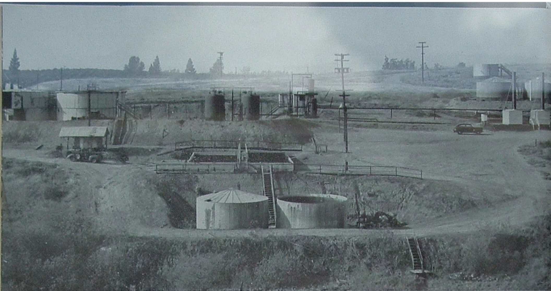
Typical of flow-line electrical dehydrator units that handle water separation in the Brea District is the above Hole Lease installation.
