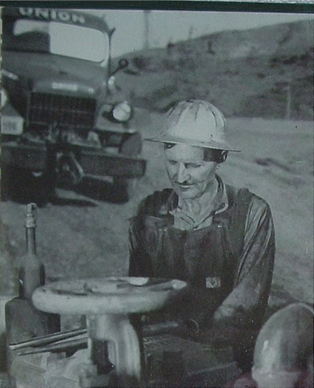
Field Mechanic A. C. Myracle, at right, tightening packing on a waste-water pump, is one of several employees who handle dehydration plant repairs in the Brea District.
