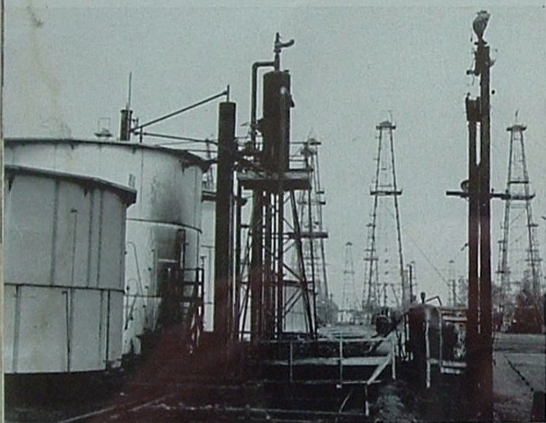
Amid a Santa Fe Springs forest of oil derricks, this unit employs the chemical "Tret-O-Lite" to separate some 14,000 barrels of water from 4,000 barrels of dry oil daily.
