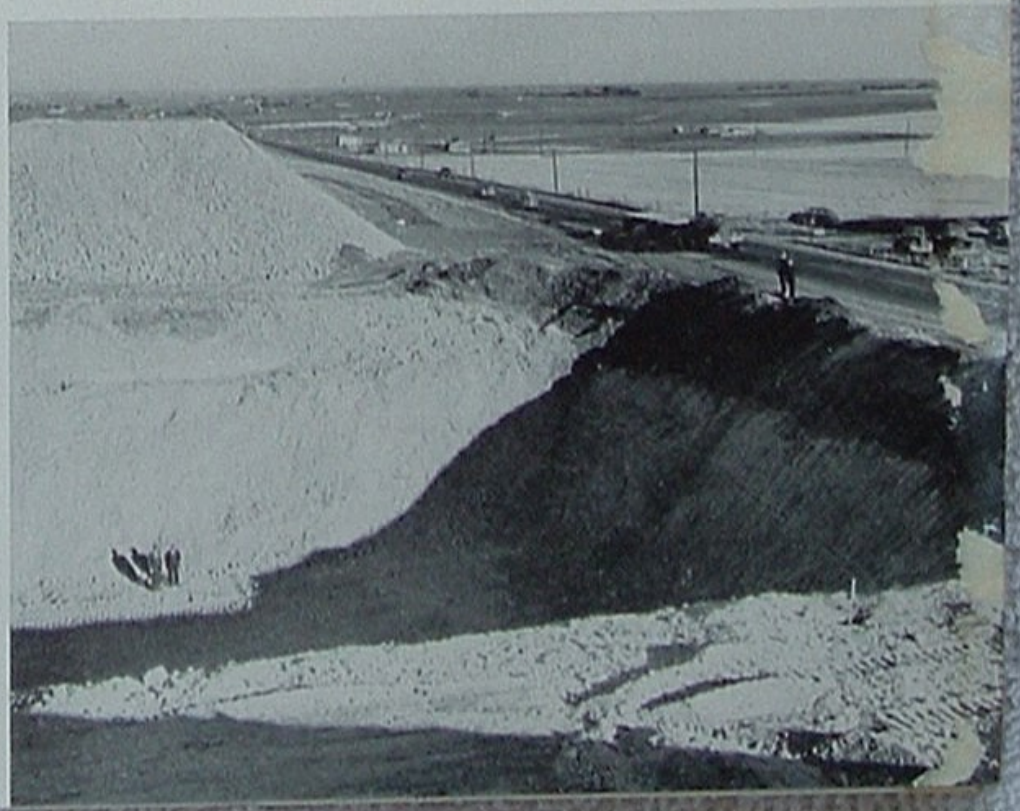
Two men standing in the excavation give an indication of the canal's proportions. Its lined trough will carry 4,600 second-feet of water.
