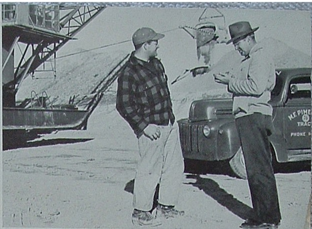
Consignee M. F. Pimentel, right, commits Engineer Arthur Gray's oil order to writing to assure faultless service and a complete supply of Company products on the Delta-Mendota Canal job. The mammoth dragline excavator, below, holds a 15-yard bucket on its 200' boom.
