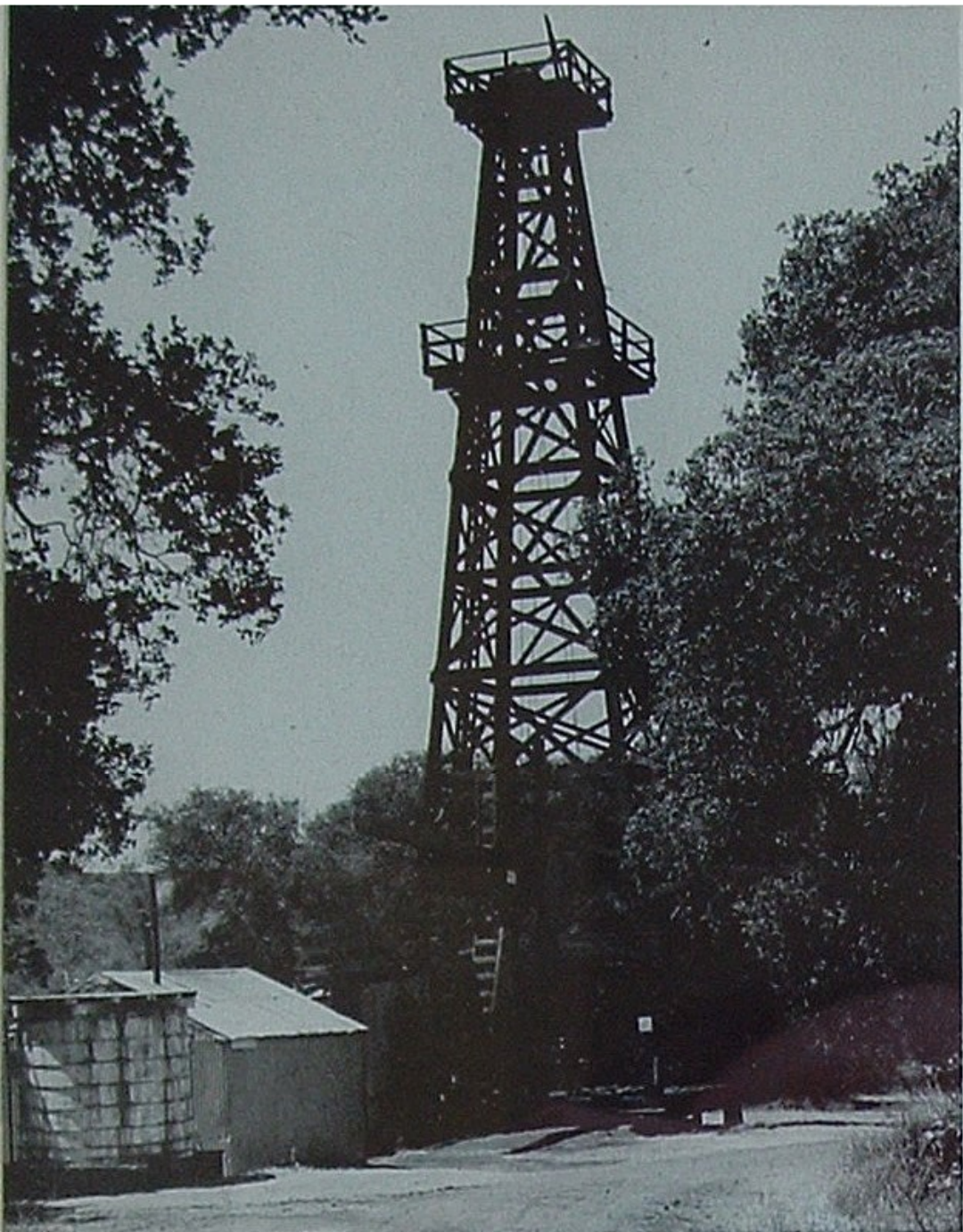
Last of our wooden derricks in the Orcutt district, this veteran of 1906 has bowed to progress and the age of steel rigs.
