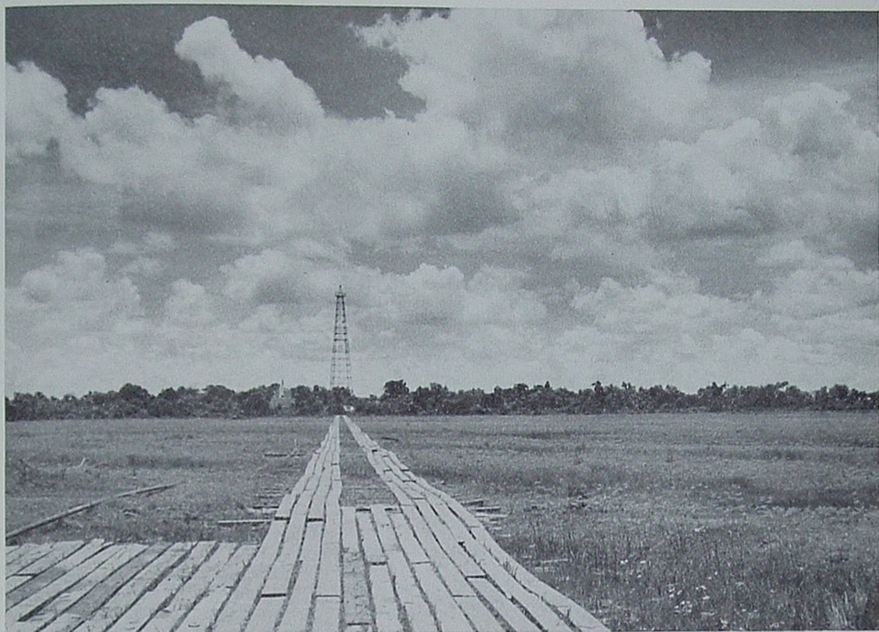
This is a Company well in the Vinton Field of Louisiana. The meadow-like foreground is actually a quagmire of silt and water, necessitating a plank road for the movement of even the lightest vehicles. Balloon-tired "swamp buggies" are used as pick-ups.
