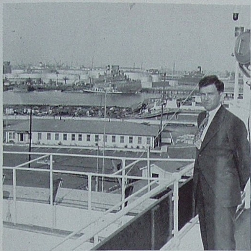
Second Mate William H. Thompson (above), stood in about this location aboard the ST. CLAIR when the MARKAY (background) exploded.
