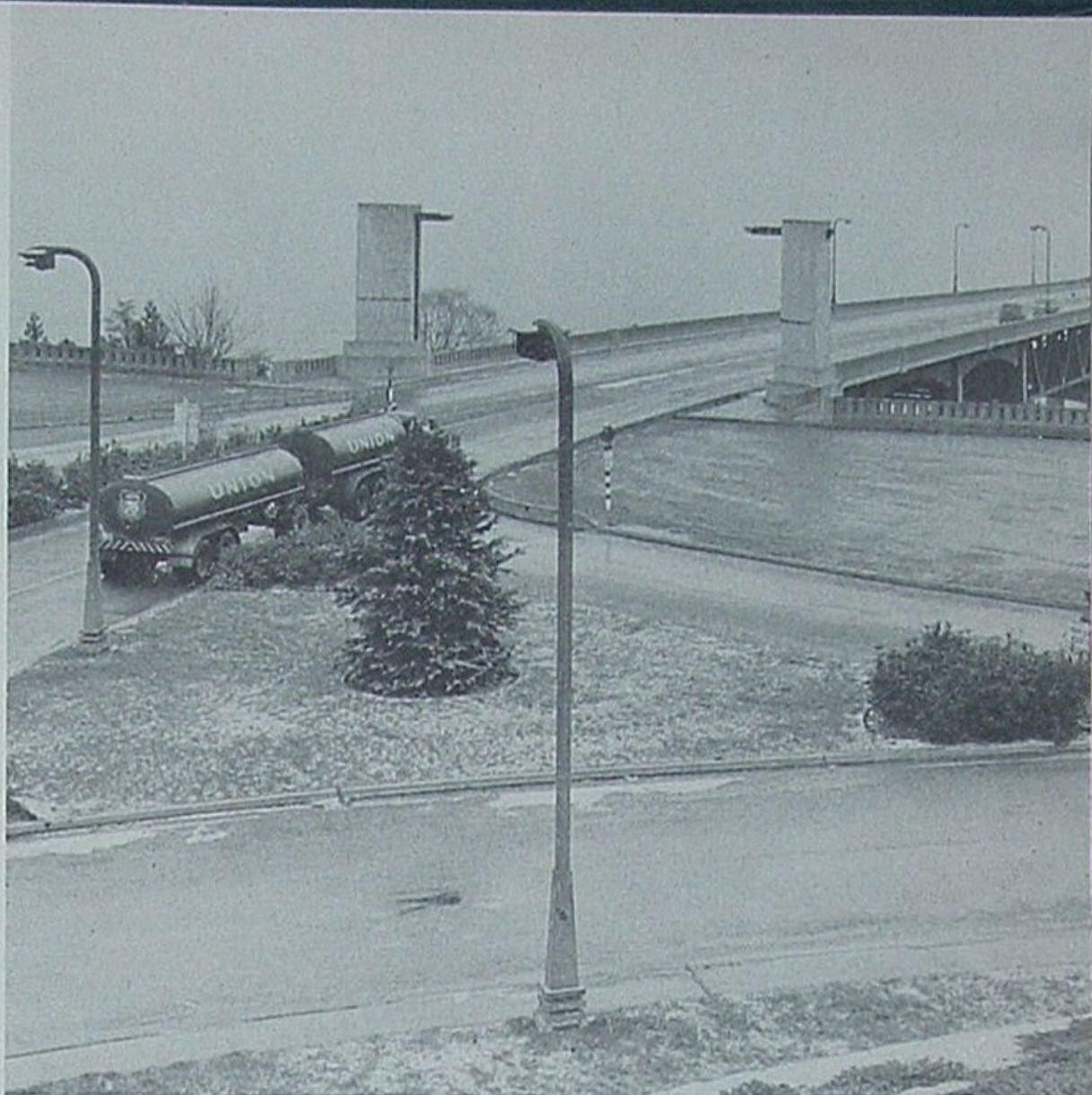
WORLD'S LARGEST FLOATING BRIDGE across Lake Washington frequently accomodates Union transports bound for points east of Seattle.
