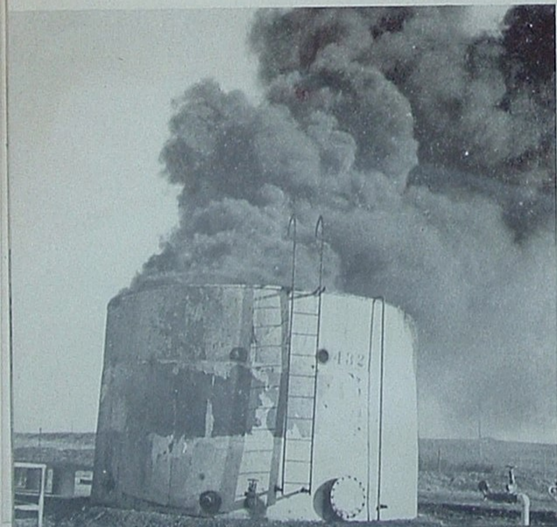
Our San Luis Obispo training grounds boasts this storage tank facility. Such contained fires are fought successfully with chemicals that form a smothering barrier between oil surfaces and the air.
