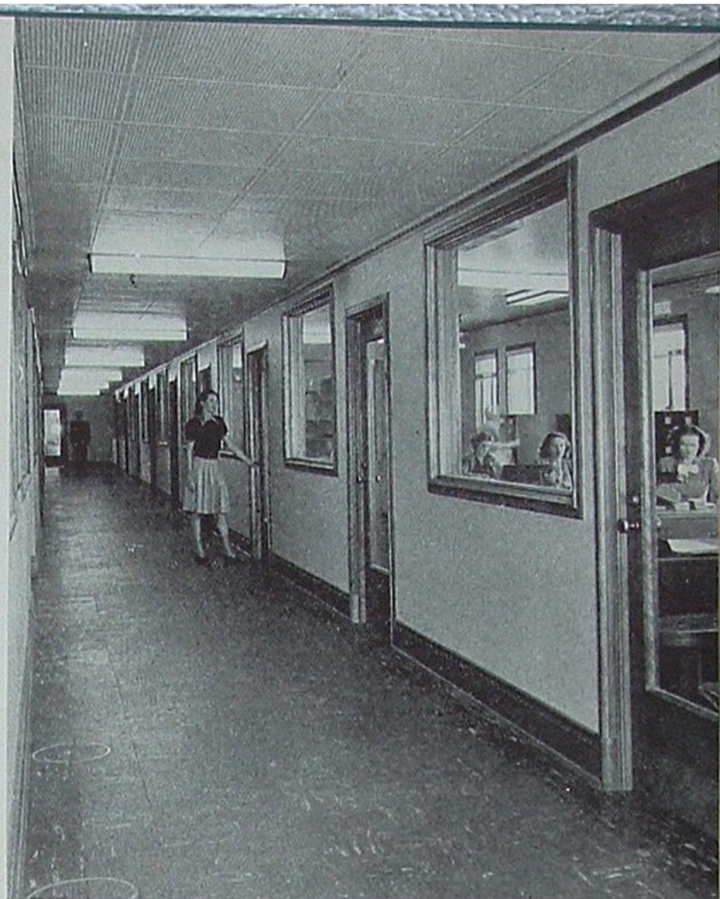
Administration Building has space for 102 single offices. Some have been combined, as in the case of Payroll. Note the interior windows, sound-proofed ceilings. Floor is of special sound-deadening construction.
