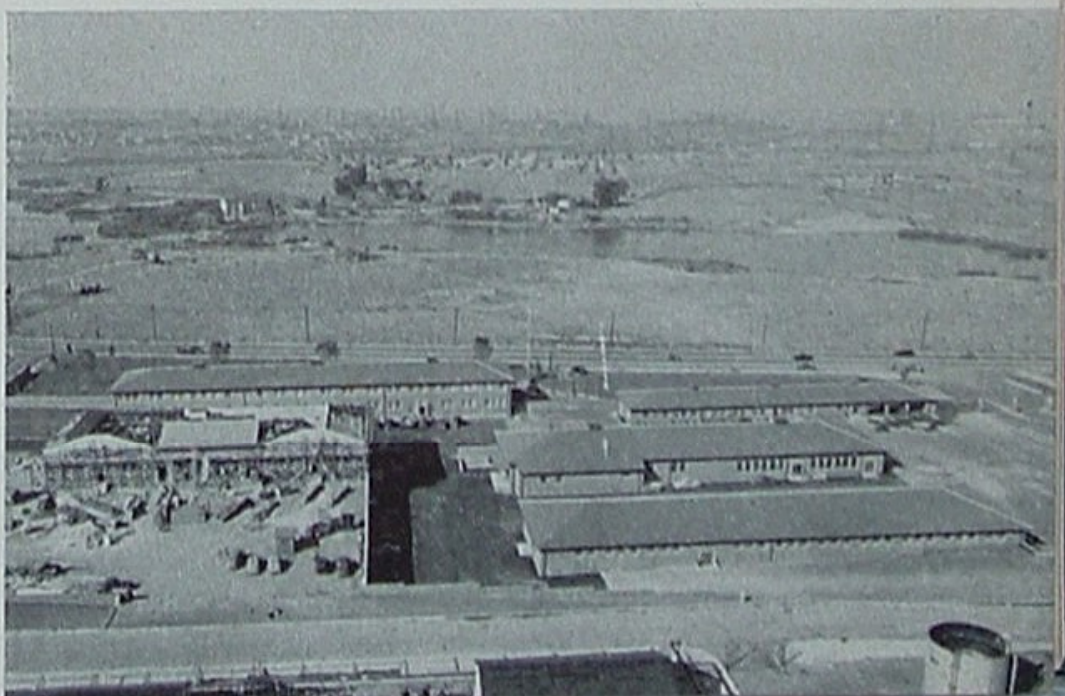
View from atop the TCC: All of the buildings are completed or occupied except the Laboratory (Left). As a safety measure, storage rooms in this building are equipped with automatic doors, sprinklers.
