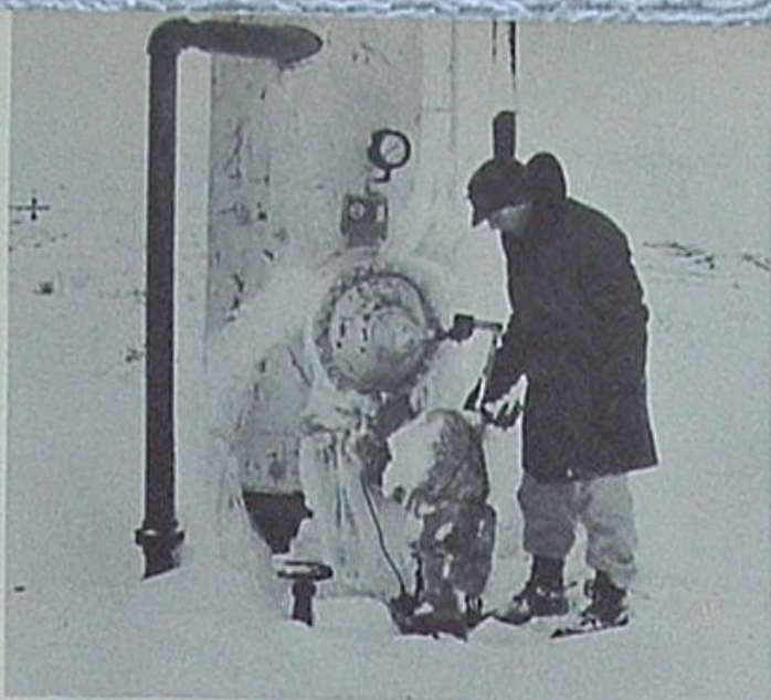
Jim Watson, Production Superintendent, is checking the float arm on a partially frozen gas trap. Jim was assaying storm damage.
