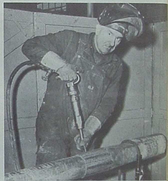
Practically all repair work for field and refinery is done in the Company's own shops. Here, Bill Reyman is peening a weld on a 6" drill collar.
