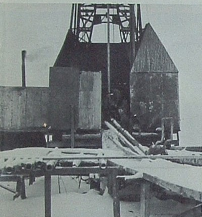
California and Louisiana roughnecks please note! This contractor's crew at Stufft No. 417-1 are running in a single.
