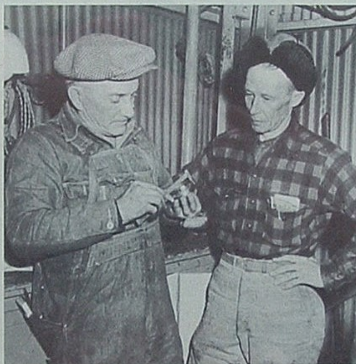
Electrician Bogi Ormson is calipering a bearing while S. and M. Sup't Leonard Shryock kibitzes. Shry's cap and shirt are vivid traffic-stoppers.
