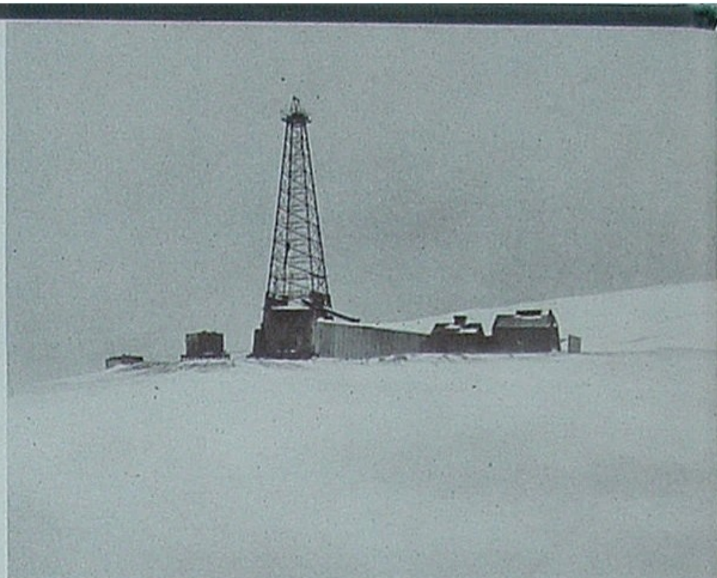
Bleak sky and snowy foreground merge in this photograph of a recently completed well in the northern part of Cut Bank Field. Like most of the other producers in the area, it was drilled with cable tools.
