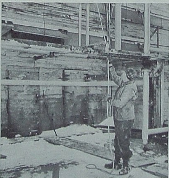
Mike Ward is opening a shutter on the absorption plant cooling tower. The shutters keep icy winds from freezing water in the tower.
