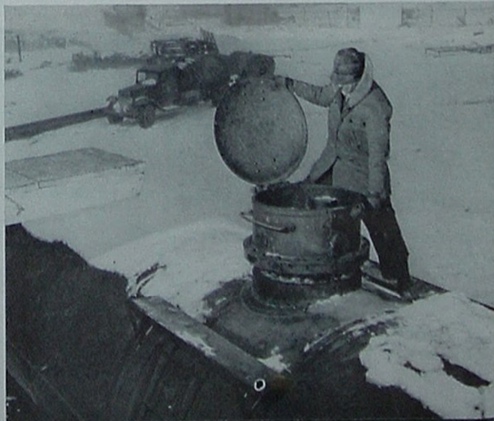
There was a blizzard blowing when this photo of a tank car loader (posed by Vern Owen) was taken. The car hauls liquified gases which are sold principally to farm accounts. (Apparent sunlight caused by flashbulb.)
