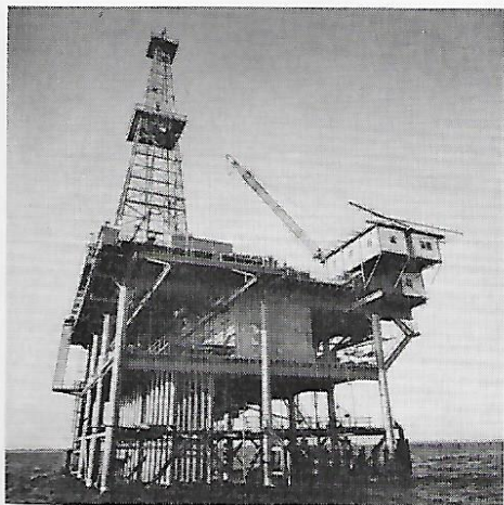
▼ "Platform Eva" off Huntington Beach, California, was the site of one of the Company's recent discoveries. The platform can accommodate 30 wells.
