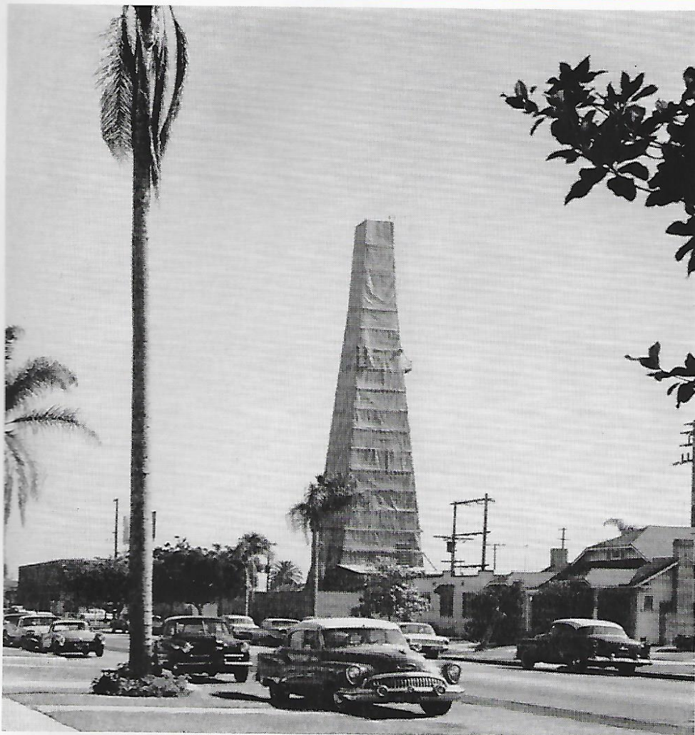
▲ This covered drilling rig is working in the Las Cienegas oil field, which covers a large section in metropolitan Los Angeles. The field was discovered by Union Oil several years ago.
