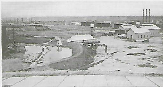
KERN RIVER PUMP STATION AND FIELD
