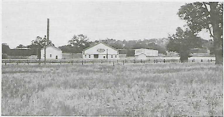
SAN LUIS OBISPO STATION FROM ROOF OF RESERVOIR
