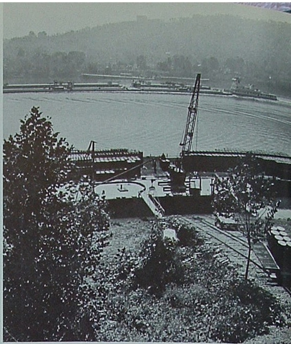
Unique inclined railway speeds barge unloading at Cincinnati.
