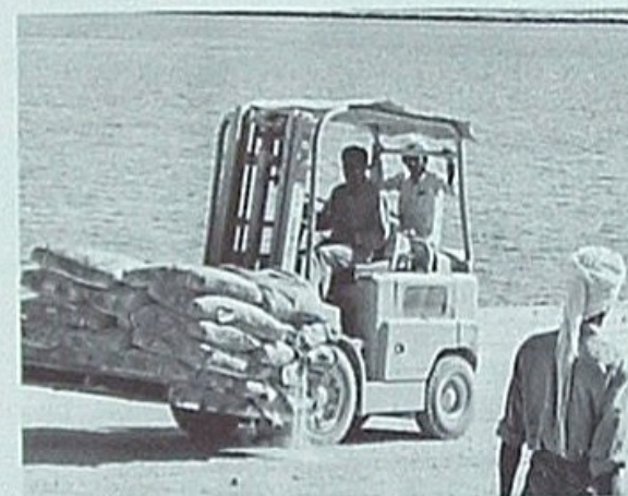
Construction workers on Lavan Island.
