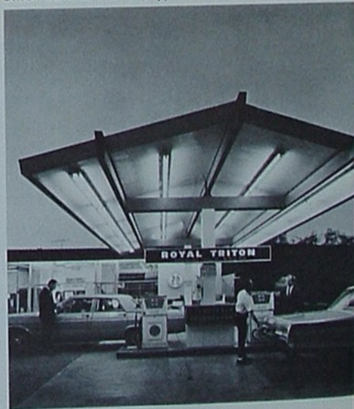
Union service station, type 300-R
