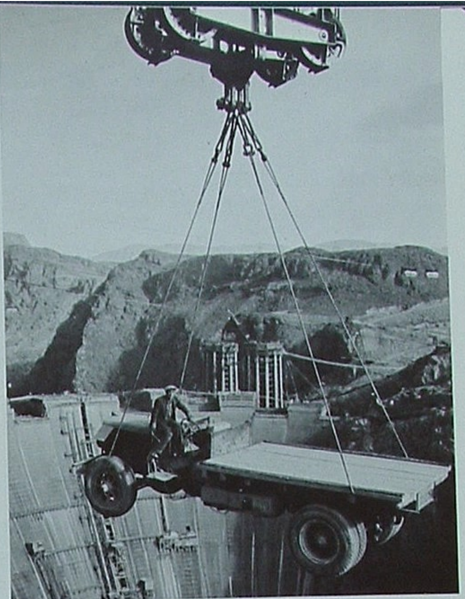
Trucks had to be lowered to canyon floor by derrick.
