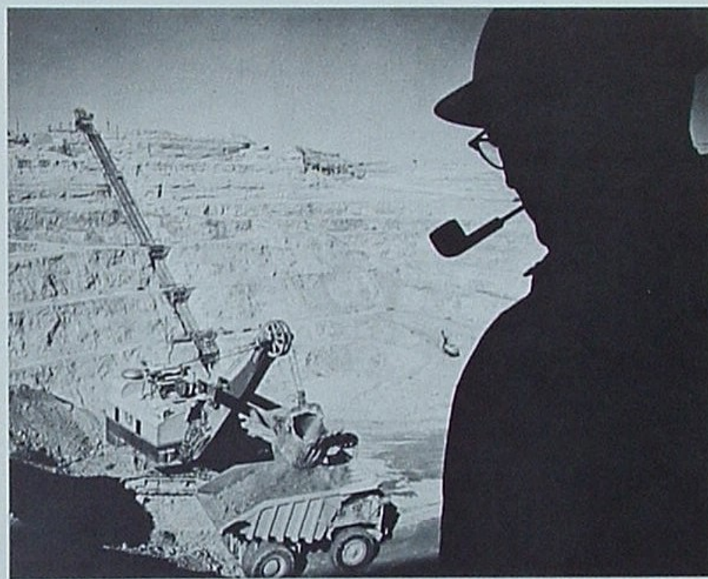
Open pit at Pima Mining dwarfs 85-ton truck and 13-ton shovel.
