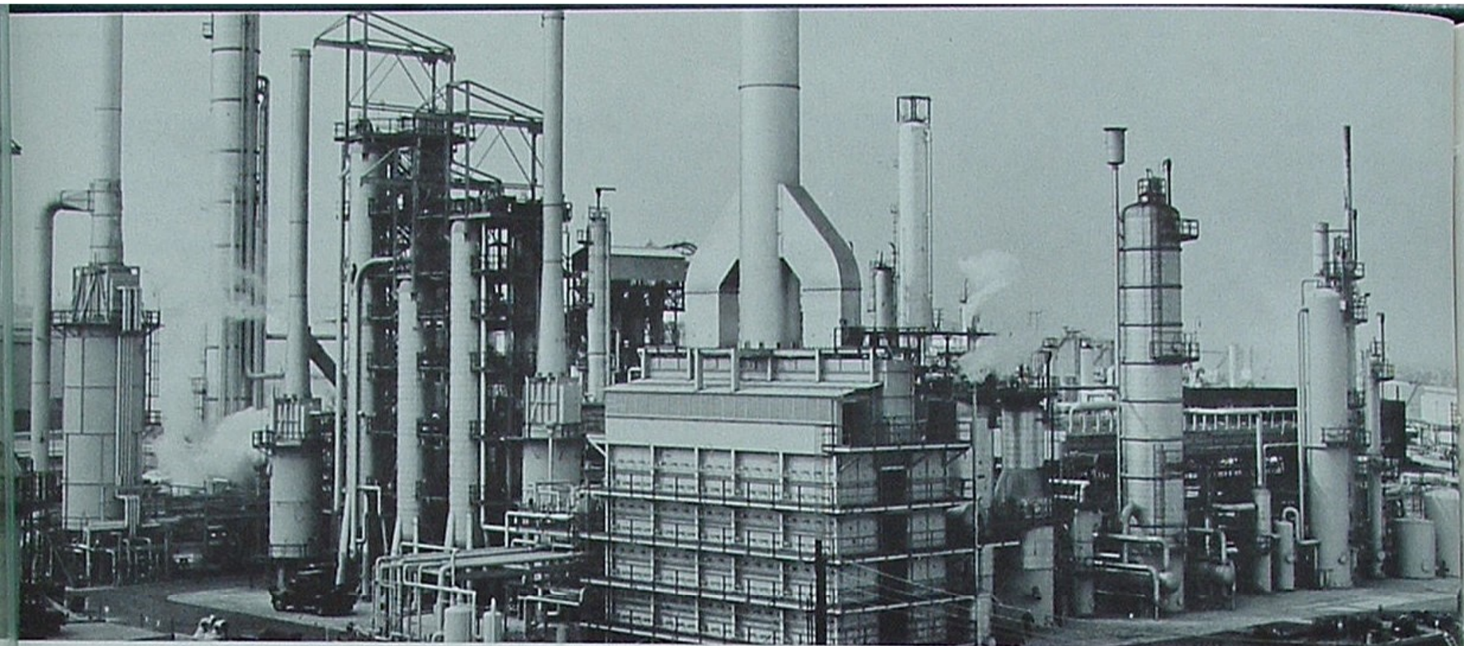
Here is the finished Unicracker, operating better than design in every respect, according to those who work with it every day.
