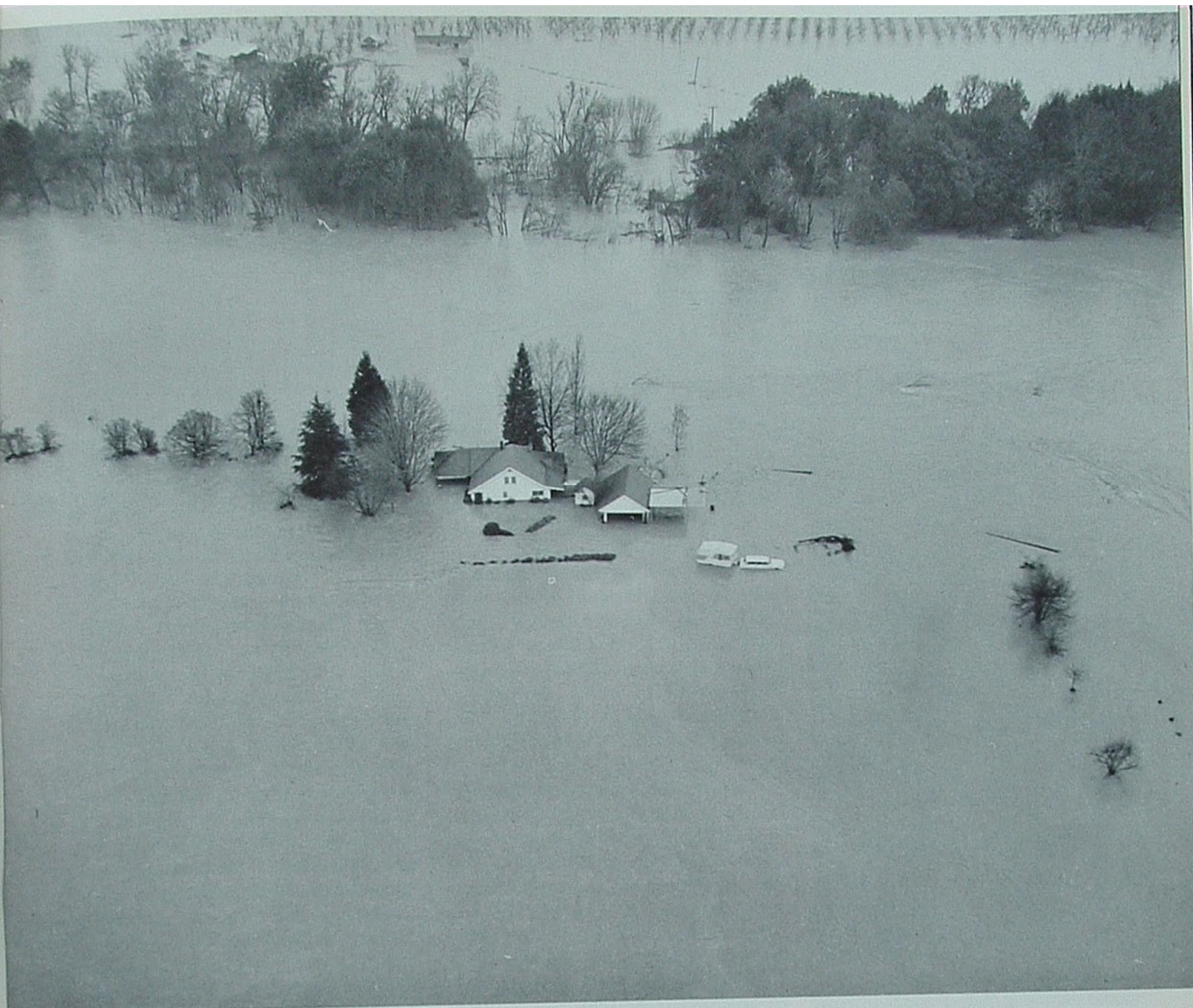
OREGON FLOODS: The countryside was a confused pattern of wet and dry areas; a few inches in elevation saved many homes.
