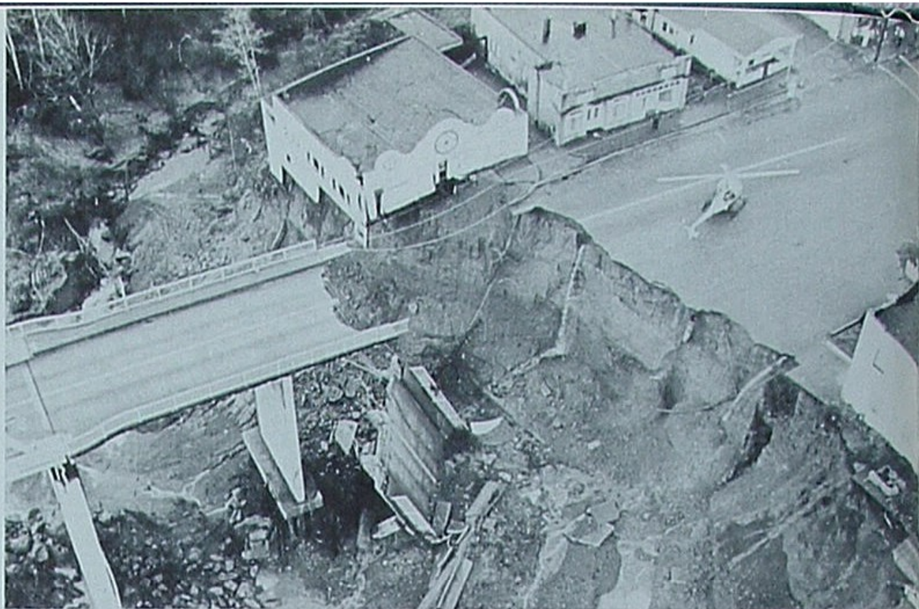
RIO DELL, CALIF: To deliver six truckloads of petroleum products across this washed out bridge, Gerald Goyan and Larry Renner used a special relay system, pumping from one truck to the other across the span.
