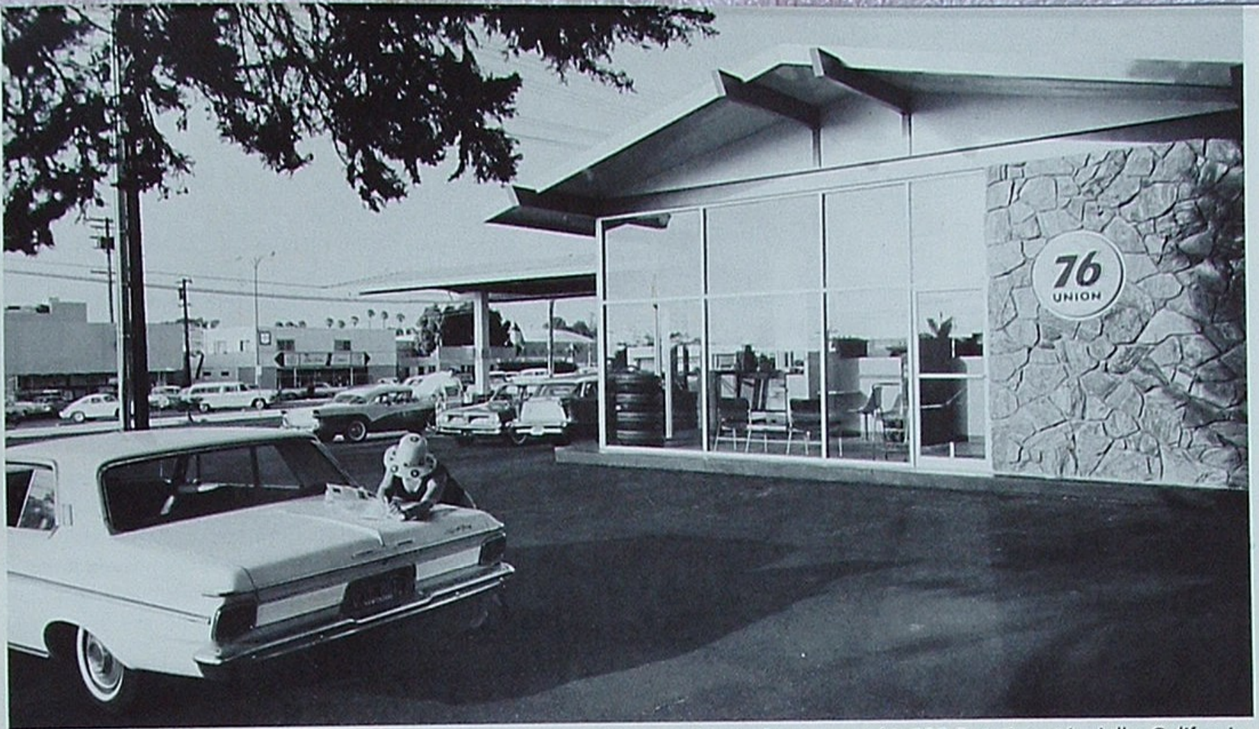
Pitched roof, showcase sales room, rock veneer wall and aluminum sash storefront grace this 300-R station at La Jolla, California.
