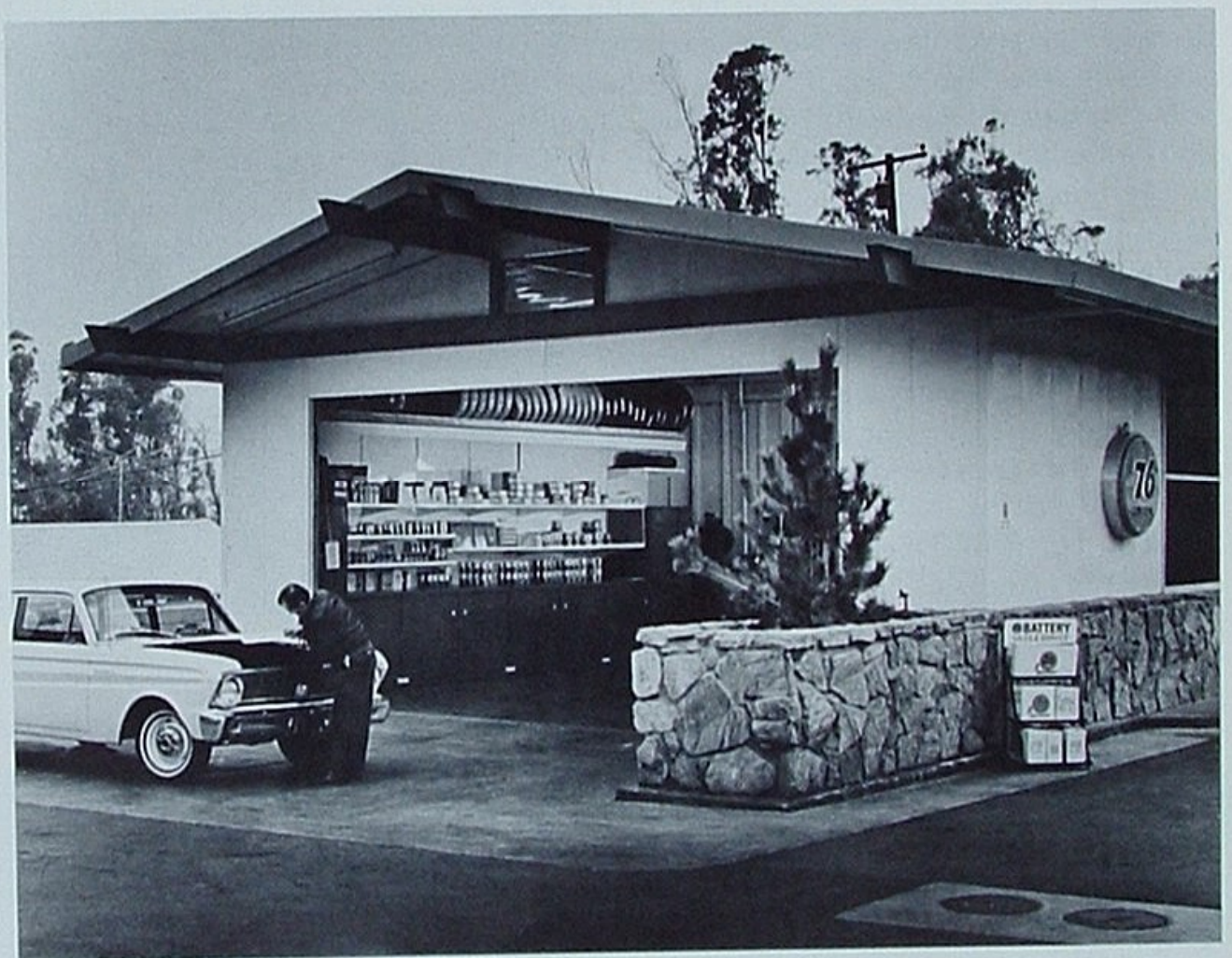
Entrance to lube room is situated at rear of Paul Lindberg's station in El Modena, Calif. Storeroom is eliminated; accessories are displayed on open shelves in lube room.
