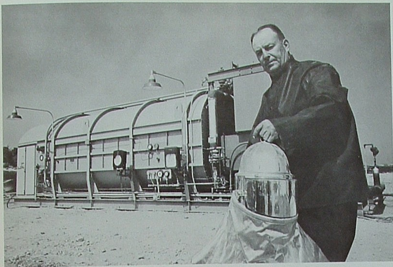
THERMAL PORTRAIT: Operator Richard J. Penny of Guadelupe poses in front of skid-mounted thermal unit. Fuel is natural gas. Steam generator has rated capacity of 17,500 pounds of saturated steam an hour.
