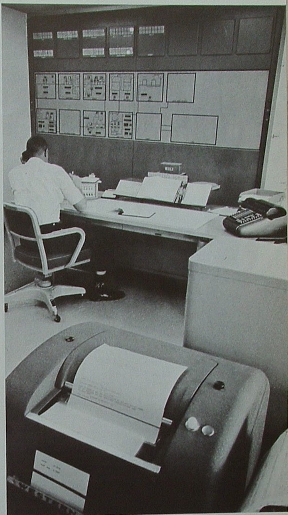
DISPATCH CENTER: From this electronic control board in Union Oil Center, two pipeline dispatchers can direct the flow of oil products, both refined and crude, throughout much of California.
