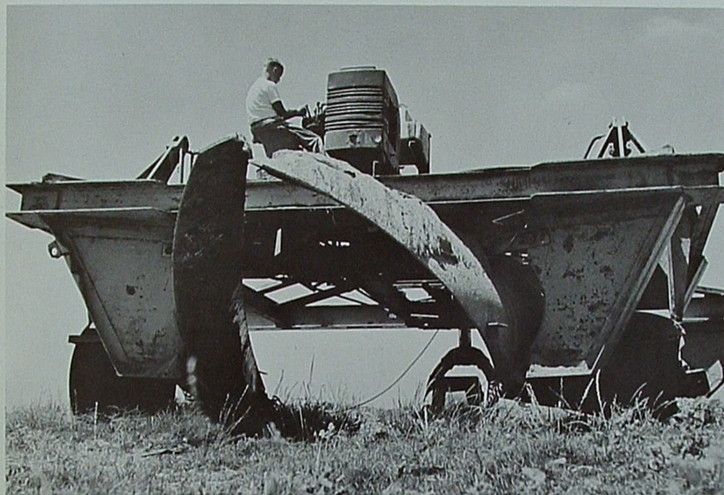
PADDY FORMER: Building rice paddies by hand was once one of the hardest jobs on the farm. This gasoline-powered machine now handles the onerous chore quickly, neatly.
