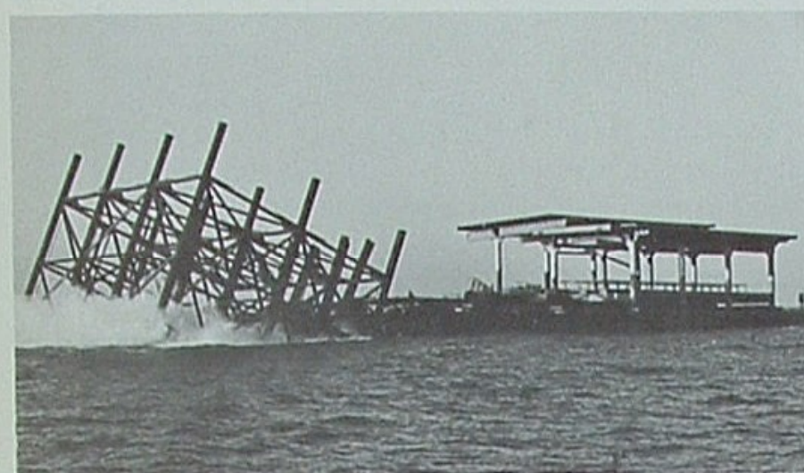
Above: The jacket, engineered to float, tipped with a Texas-sized splash. Method of installing is described in the article.
