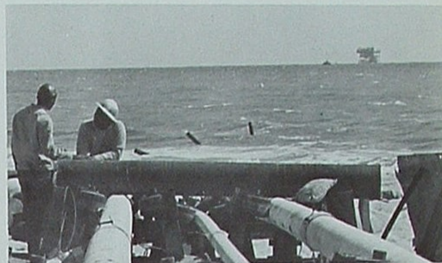
Top: Derrick barge lifted decks onto jacket, making complete platform. Installation of equipment followed. Center: Pipelines were welded into 600 foot lengths and drawn out to platform at sea by seagoing tow-barge. Below: Union Oil began drilling from platform on May 8, even before heliport was installed.
