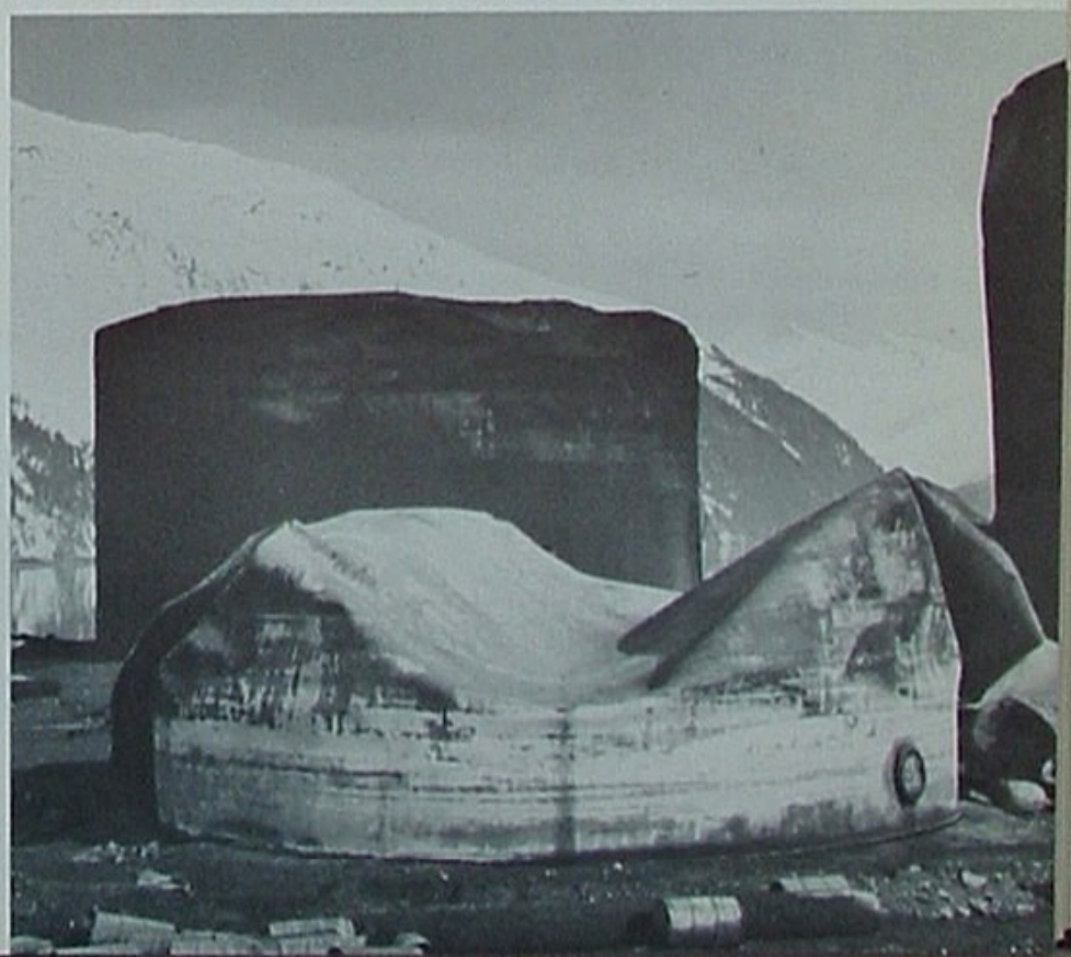
Tank at Whittier appears as if giant had stepped on it. Glaciated peaks in background are Chugach Mountains
