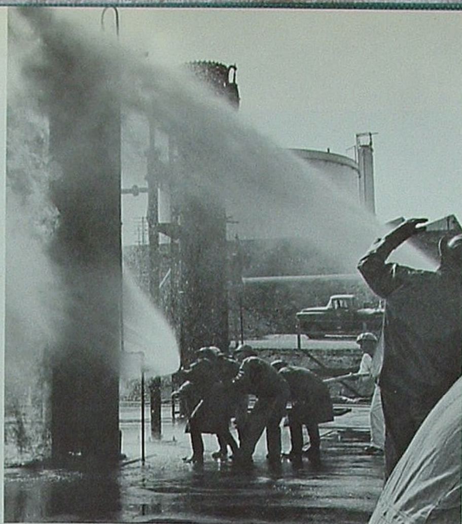
Above left, team prepares water spray attack on butane fire. Above right, first team covers the second with water spray while latter moves toward valve to stop flow of fuel oil. This is the best way to halt fire.
