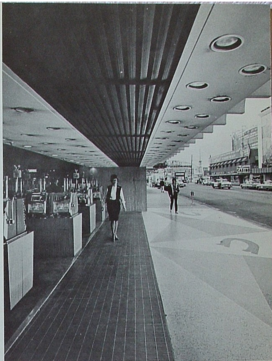
This pretty miss at the Horseshoe Club in Reno is walking through a door—an invisible door. The "air door" is a moving curtain of oil-heated (or cooled) air flowing both upward and downward through gratings. Union Oil developed a modified lubricant for filtering the air used on these casino doorways.
