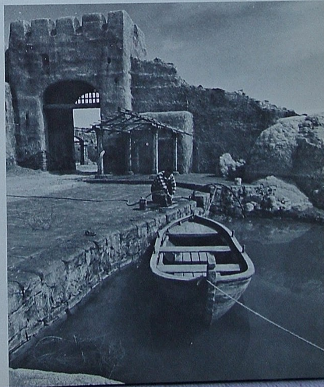
Our cameraman couldn't resist this scene of today's water carrier in checkered shirt, lifting the Sea with a gas powered pump.
