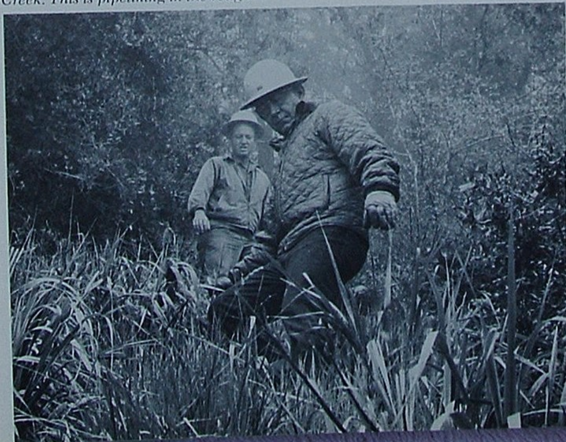
Robert Portlock and Shorty Clark (foreground) coming down the mountain at Tar Creek. This is pipelining in the rough.
