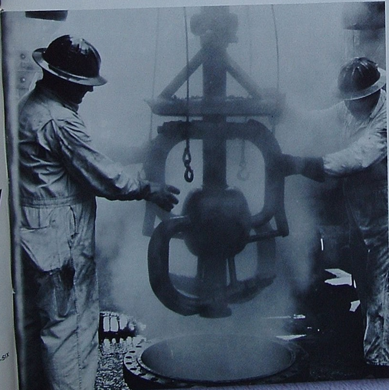
Operators atop one of the coker drums are guiding a "pretzel" down toward a pilot hole previously cut through the coke bed. This cutting tool dislodges the coke with jets of water released under 1,800 pounds of pressure.
