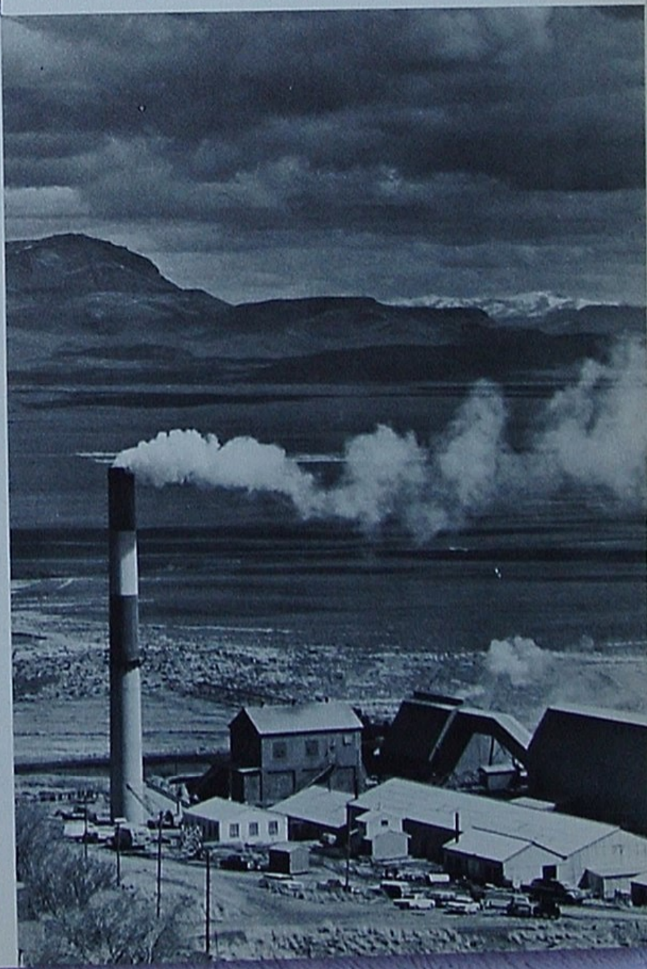
Rugged Euclid truck (left) hauls the ore and waste rock from three open-pit locations. Ore assaying a sufficiently high gold content is trucked to the mill (below) for crushing, processing and melting into bars of gold.
