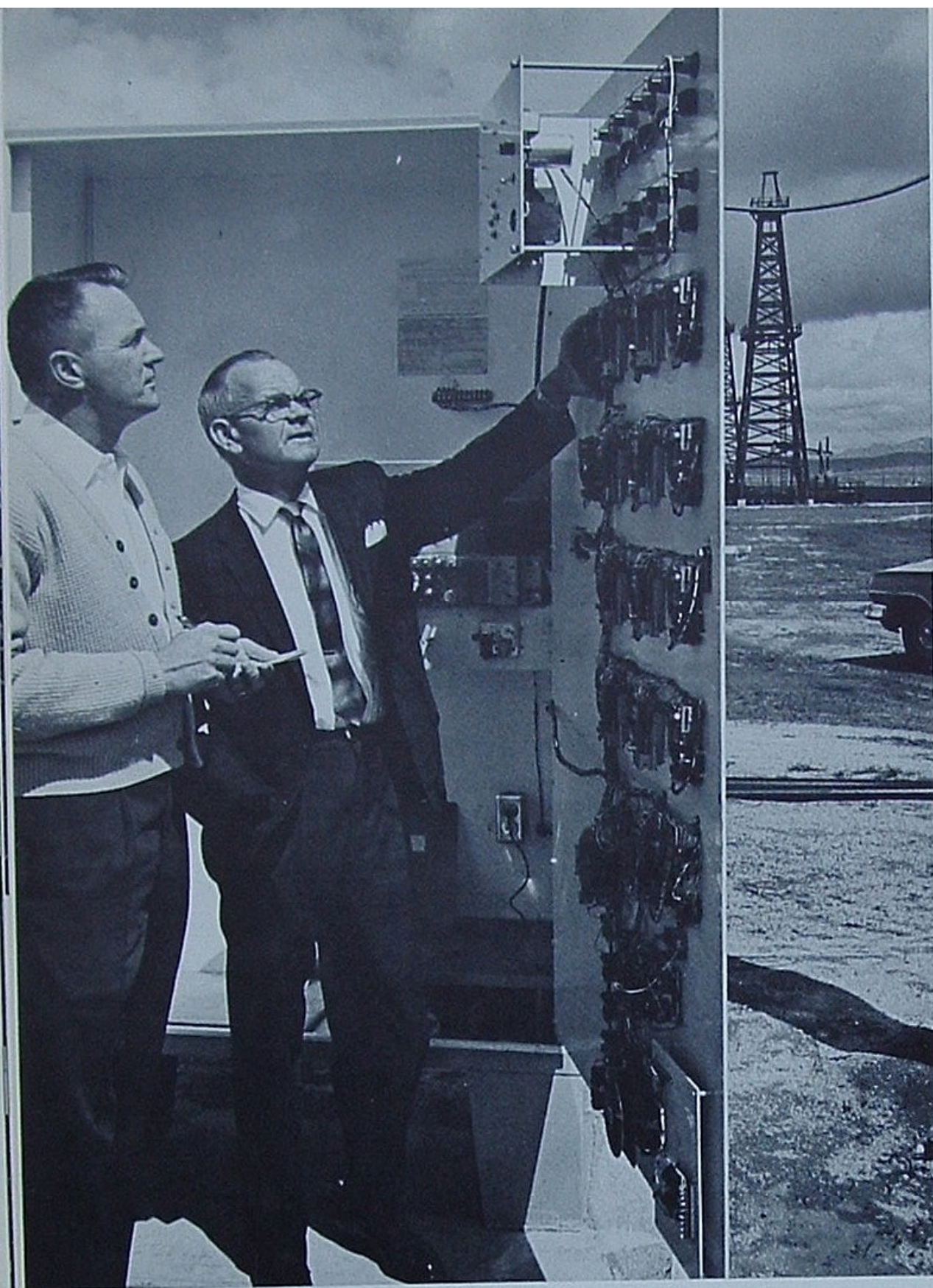
Checking final installation details with the supplier, Walter Ennis of Long Beach, is John Anderson (left), production supervisor at Bakersfield. The radio equipment relays oil measurements to Kern Station.
