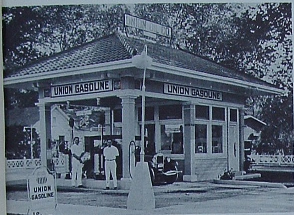
Mrs. French is adding to a Union Oil association that began nearly 40 years ago, when her husband leased this old unit.
