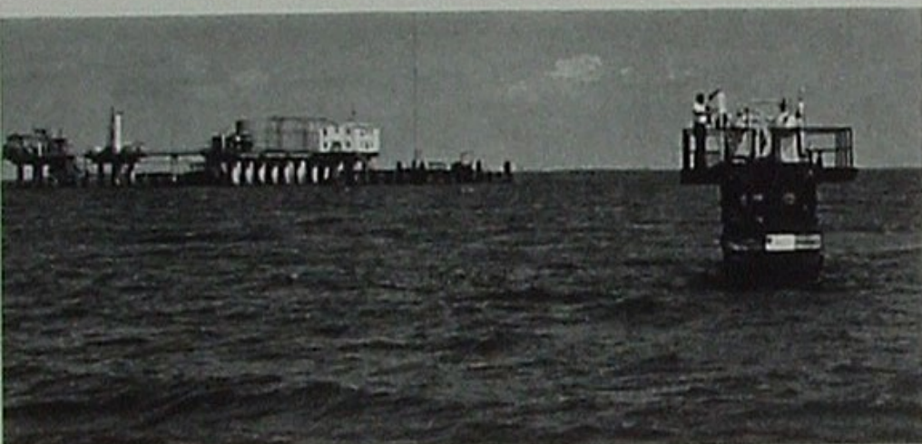
A production engineer attends ailing well.
