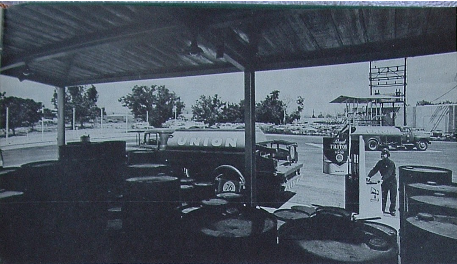
A unique feature of the new plant: covered, ground-level storage for package goods. Trucks are loaded and unloaded with power hoist.
