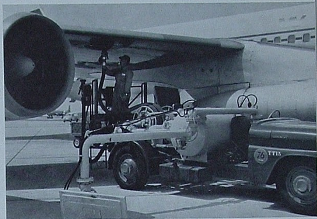
A truck is used only to effect swift hose connections between underground hydrants and airplane fuel tanks. Fast pumping rates permit fueling of jets at maximum speed.
