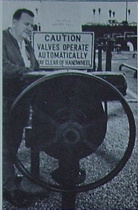
Robertson adjusts automatic valve at the L.A. Harbor pumping station.
