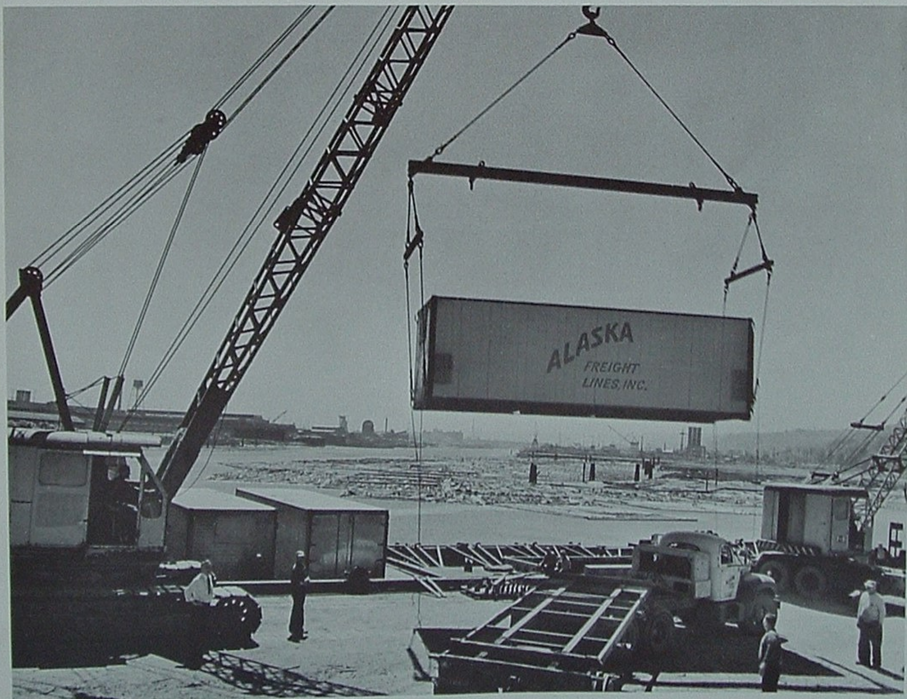
Manitowoc crane lowering 27' container on to Alaska Freight Lines skeleton trainer
