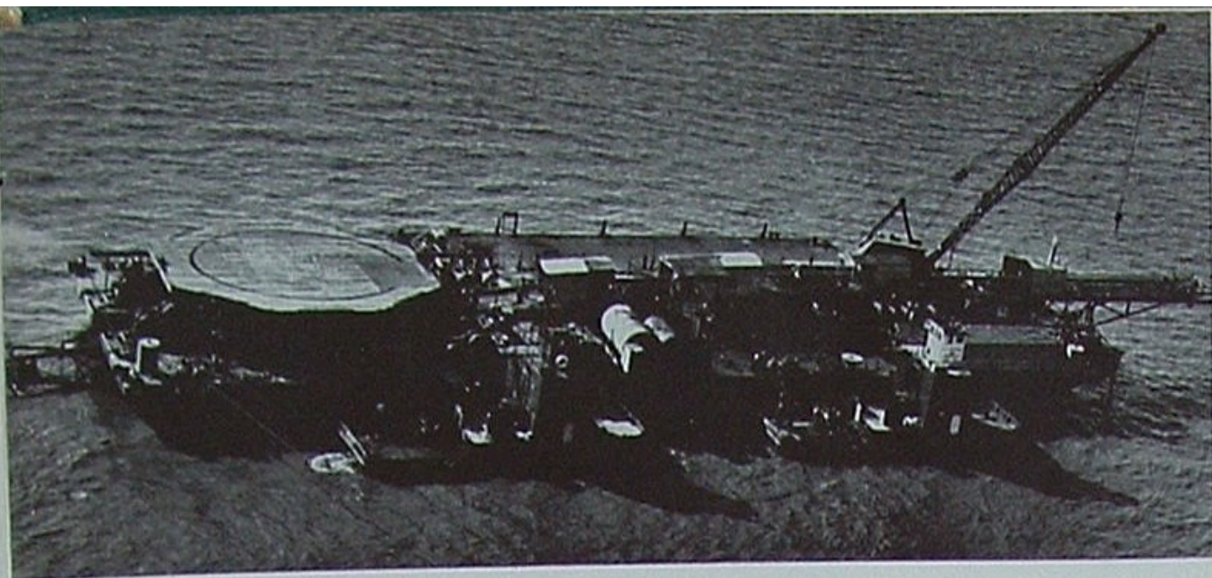
This pipe-laying barge was towed all the way from the Gulf of Mexico to get the job done. Among its built-in advantages is a helicopter deck for landing men, emergency tool orders.
