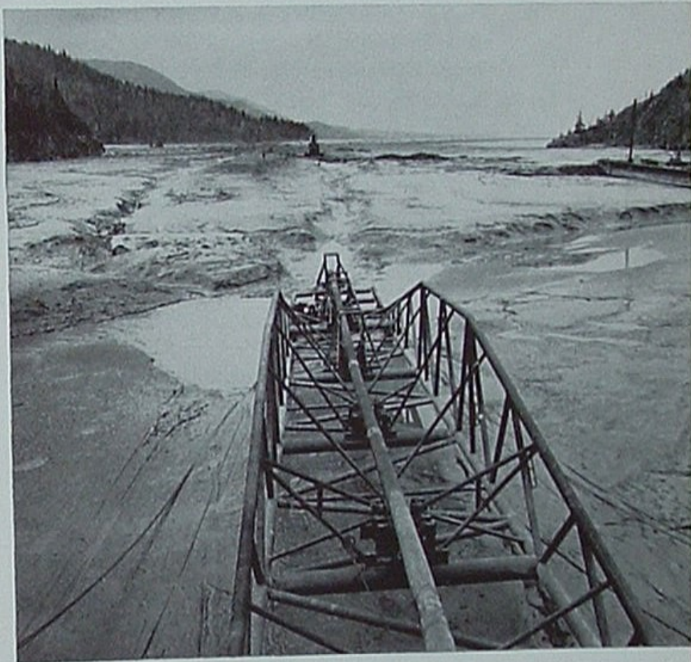
The pipe-laying "stinger" at stern of barge is seen above awaiting the return of high tide to Turnagain Arm. With the tide in, below, pipe is "put to bed" in a trench freshly dug by air and water jets, whose force boils to surface.
