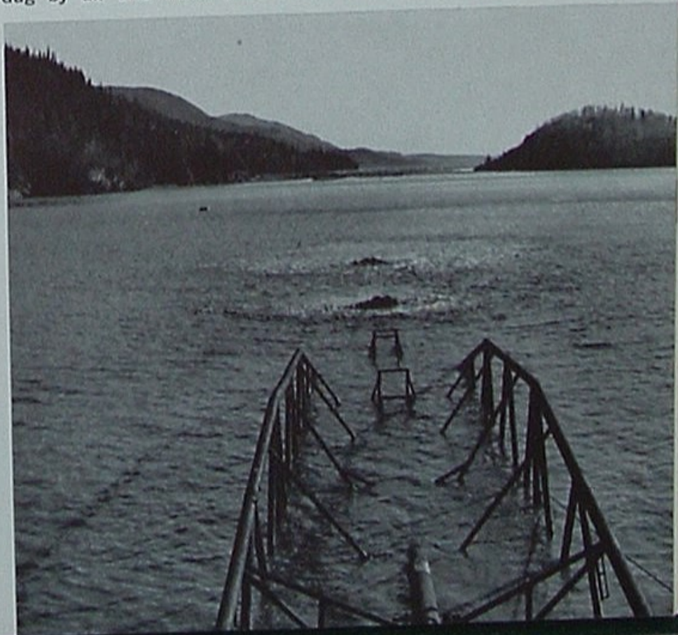
The pipe-laying "stinger" at stern of barge is seen above awaiting the return of high tide to Turnagain Arm. With the tide in, below, pipe is "put to bed" in a trench freshly dug by air and water jets, whose force boils to surface.
