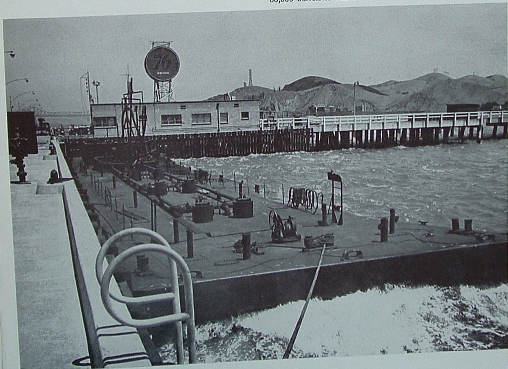
The steel barge in use at Oleum Refinery today carries a cargo of 35,000 barrels to Sacramento and return in less than 24 hours.
