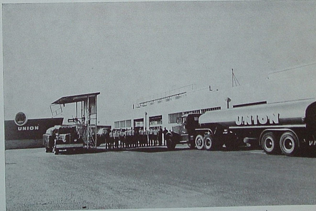
Photos of our Fresno Plant, yesterday and today, suggest some interesting contrasts: Horsepower has totally replaced horse power. With fewer vehicles and about the same number of employees, we are today supplying the Fresno city area with over a half-million gallons of petroleum a month. Fifty years ago, six tankwagons did well to deliver 2,500 gallons in a 10-hour working day.
