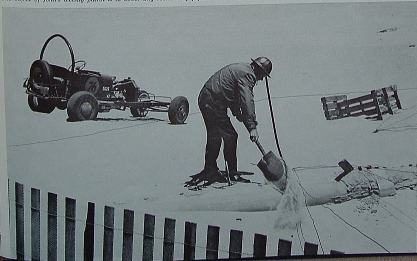
The object of John's weekly patrol is to cover any sections of pipe exposed by wind. Here even a snow fence failed to halt shifting sand.
