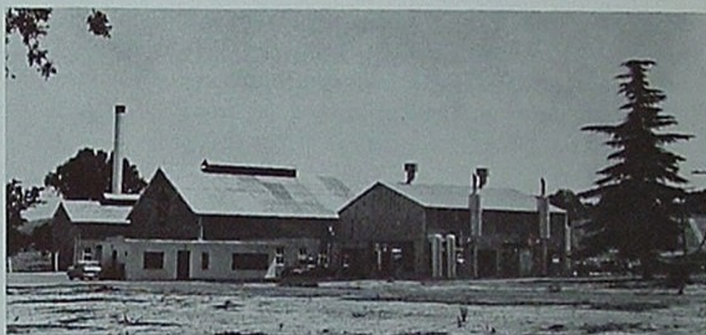
Santa Margarita is a manned pump station where oil is pumped both to and from the coast. The operator reports to Los Angeles every two hours.
