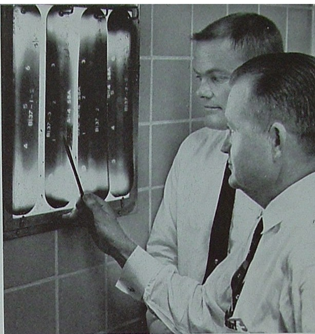
Radiographs taken of each weld tell Supervisor J. T. Patrick, right, and Metallurgical Engineer George Moller whether there are any welding imperfections between the sections of pipe.
