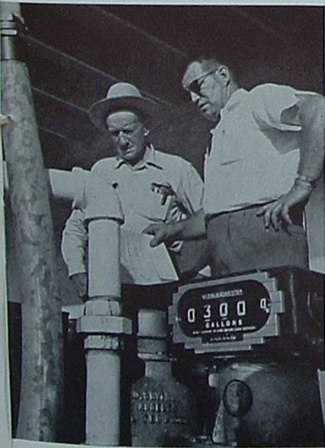
The consignee and Union Oiler Jim Luzedder "get the hang" of plant's new loading rack.
