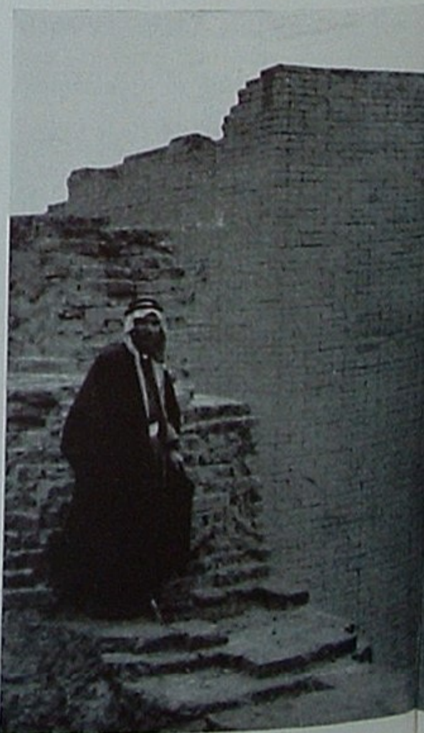
Brickwood of ancient Babylon, preserved with asphalt mortar even to this day.
