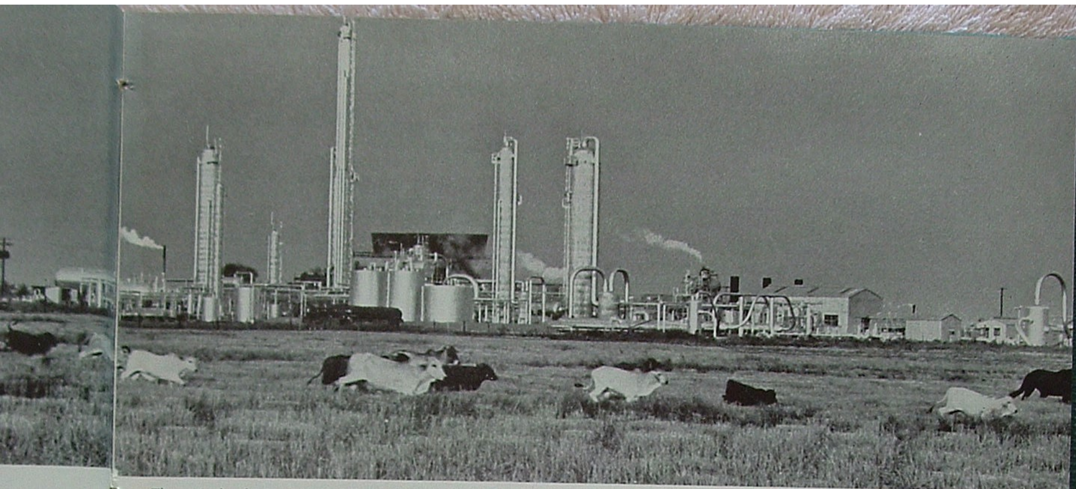
These are the shining towers of the Goliad-Union Cow Island extraction plant. The plant recovers valuable liquids formerly left in natural gas sold to interstate pipelines to be burned as fuel. There's no doubt where this island location got its name!
