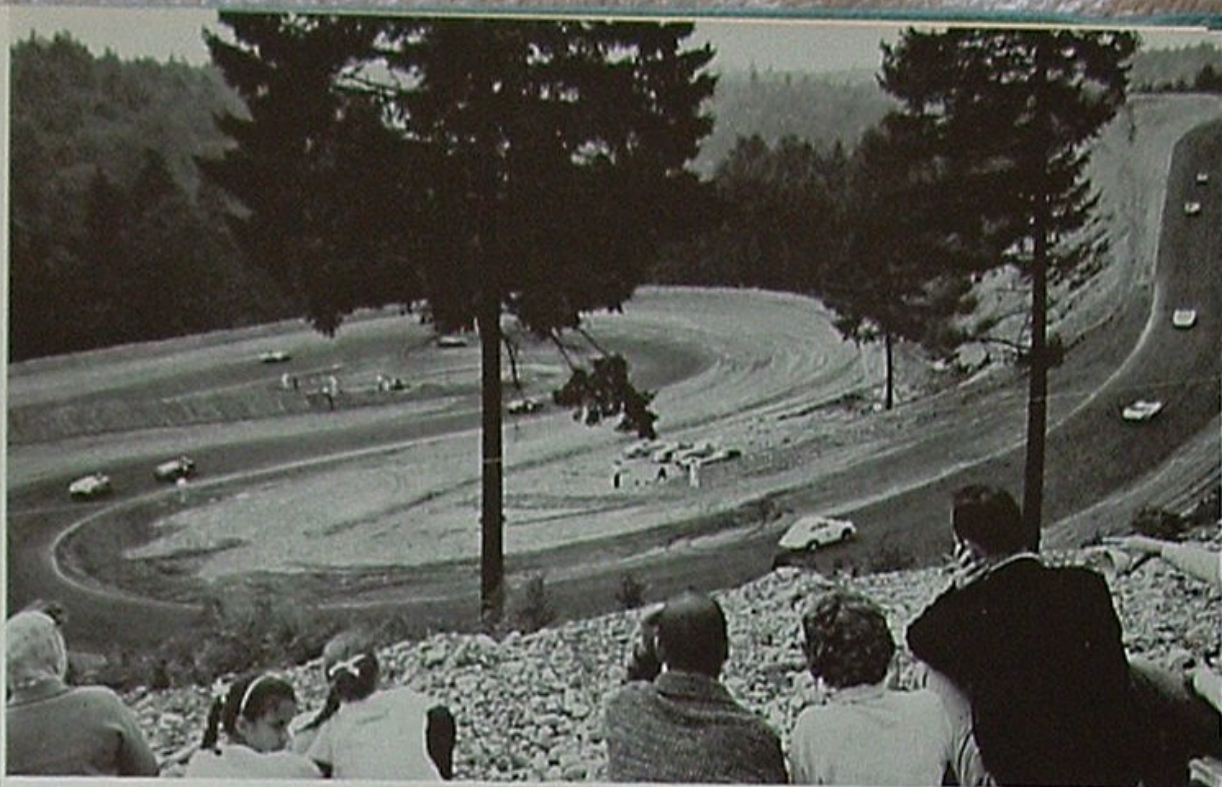
Viewing and safety advantages were achieved by locating the track's S-curve beneath spectator location on a hilltop.
