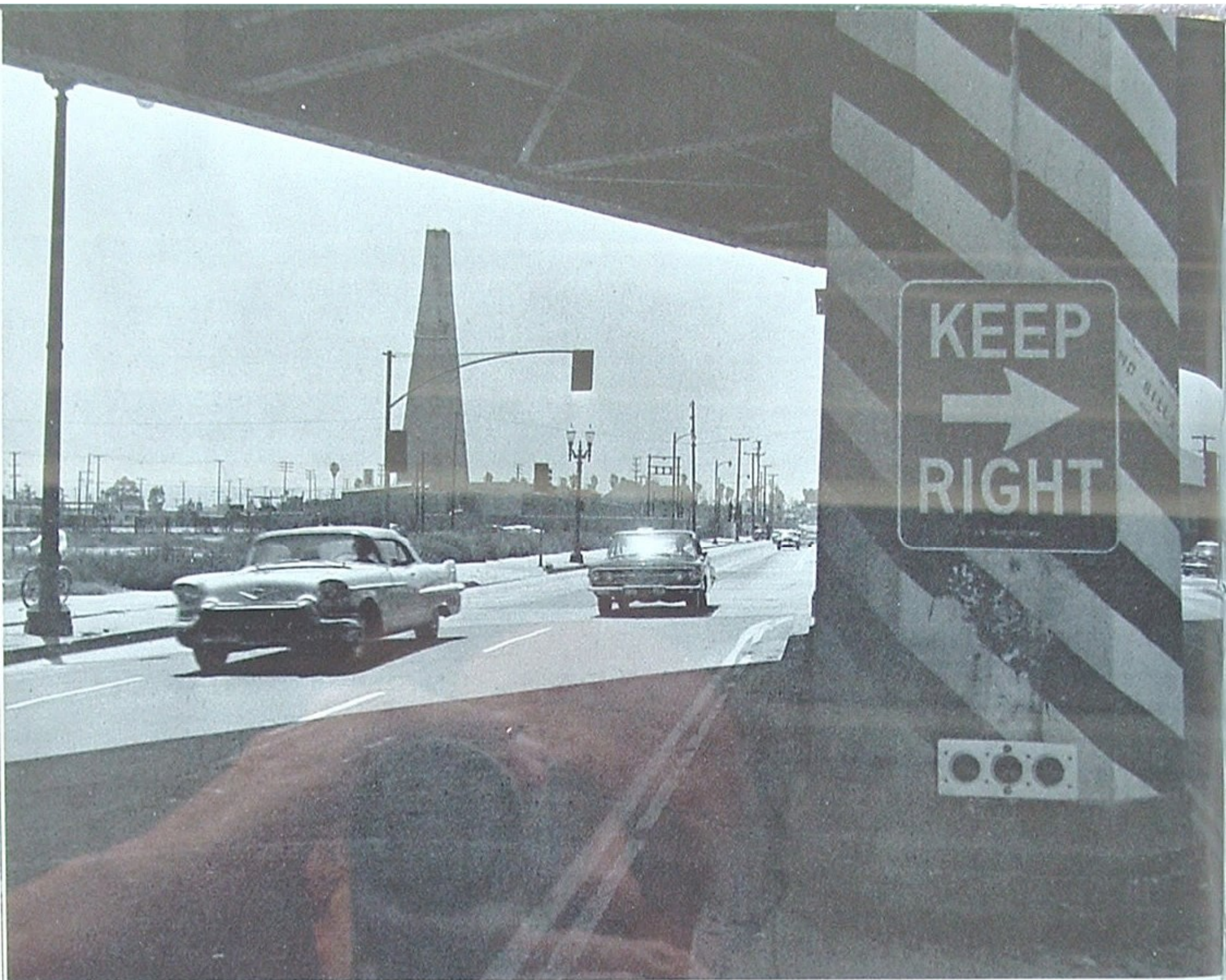
Inside its "poke" of soundproofing, this Union Oil exploratory well has opened a new oil field in one of the busy parts of Los Angeles.
