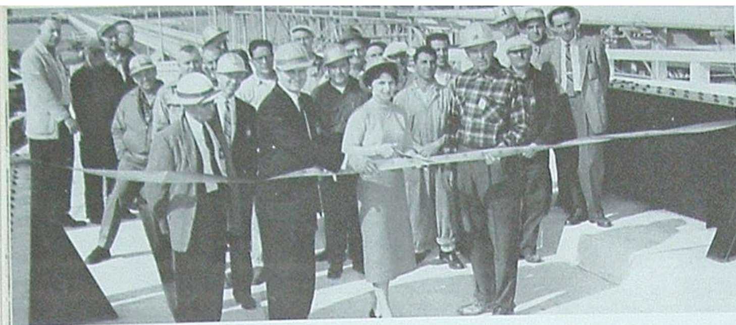
LAVONNE O'NEAL, secretary to the manager of Oleum Refinery, was chosen as official ribbon cutter at the opening on March 30 of a new concrete-and-steel access ramp to Oleum's marine terminal. The ramp replaces a wooden trestle and eliminates a grade crossing over Southern Pacific tracks.
