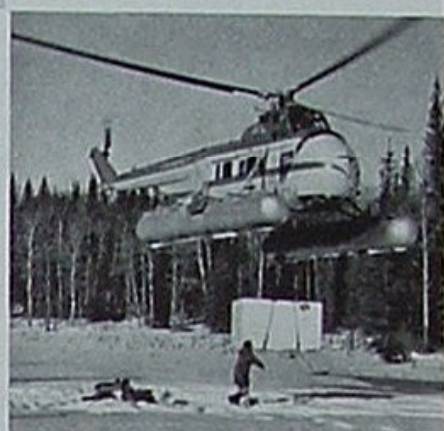
For winter seismic operations the helicopter is invaluable. The box it is carrying, above and at right, soon takes shape, below, as the recording hut.
